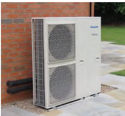
Photo 41. Air source heat pump (note the external pipework can also be visually unattractive and should be positioned carefully).
