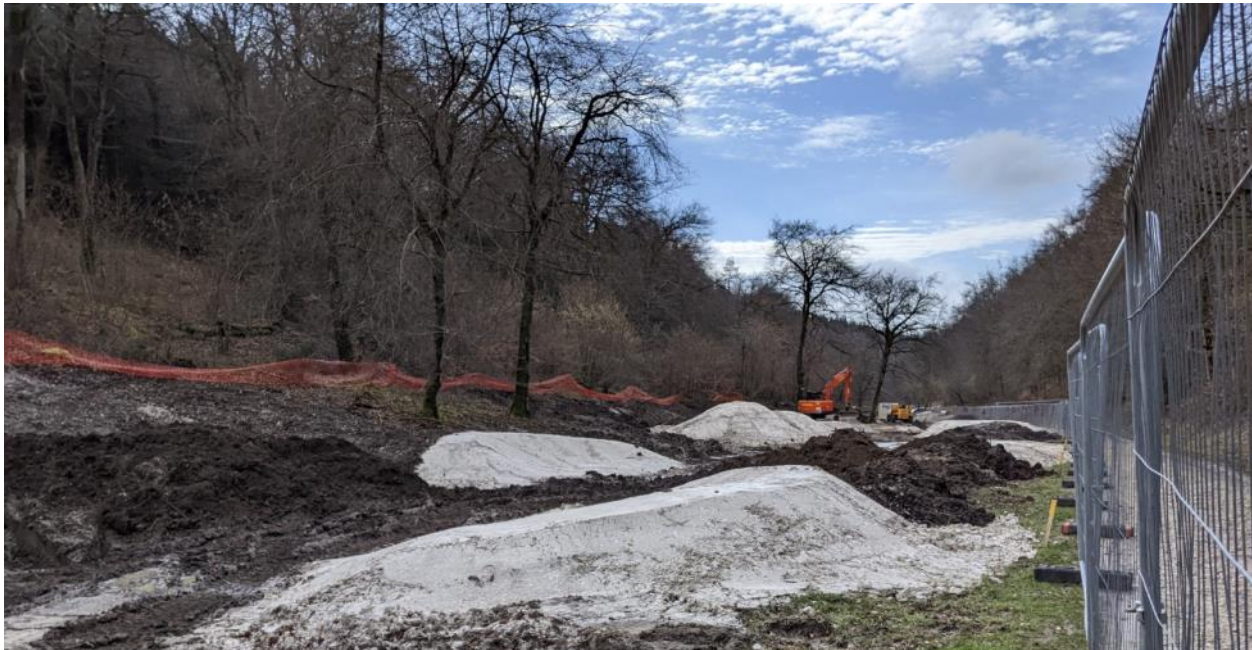
Skills area early construction (image right & below)
