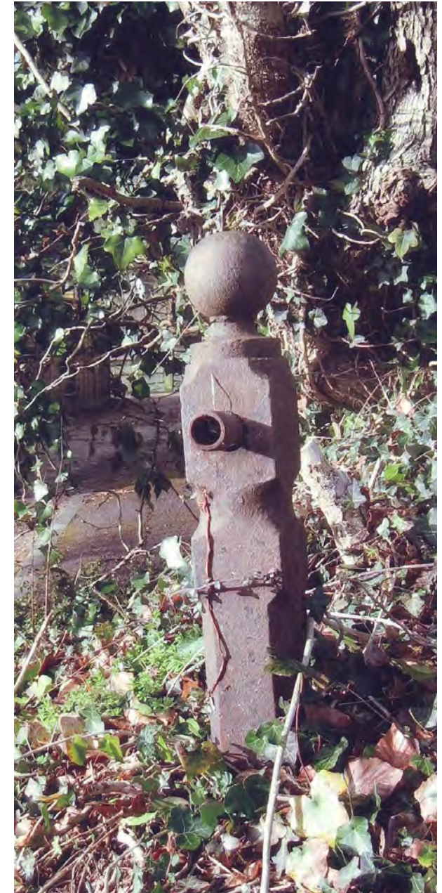
Standpipe outside Copper Beech House
