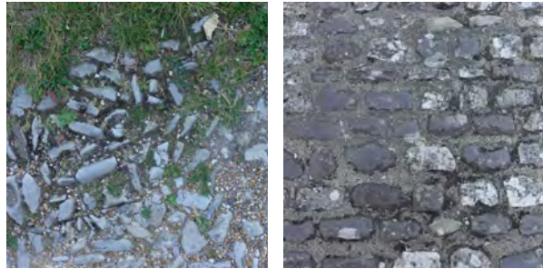
LEFT: Cobbles in front of the Old Butchers Shop RIGHT: Blue ragstone path in front of the Gallery
