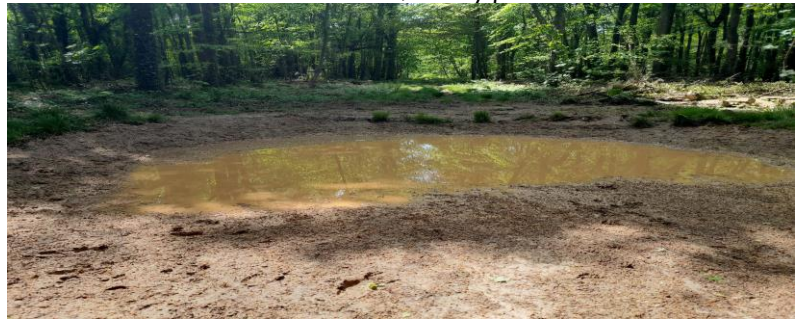
Wetted Bentonite, forming the clay liner
