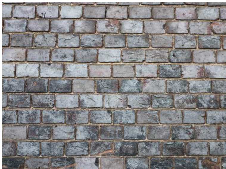
Figure 50: Grey brick headers. On close inspection the red undertones of the brick can be seen beneath the grey finish
