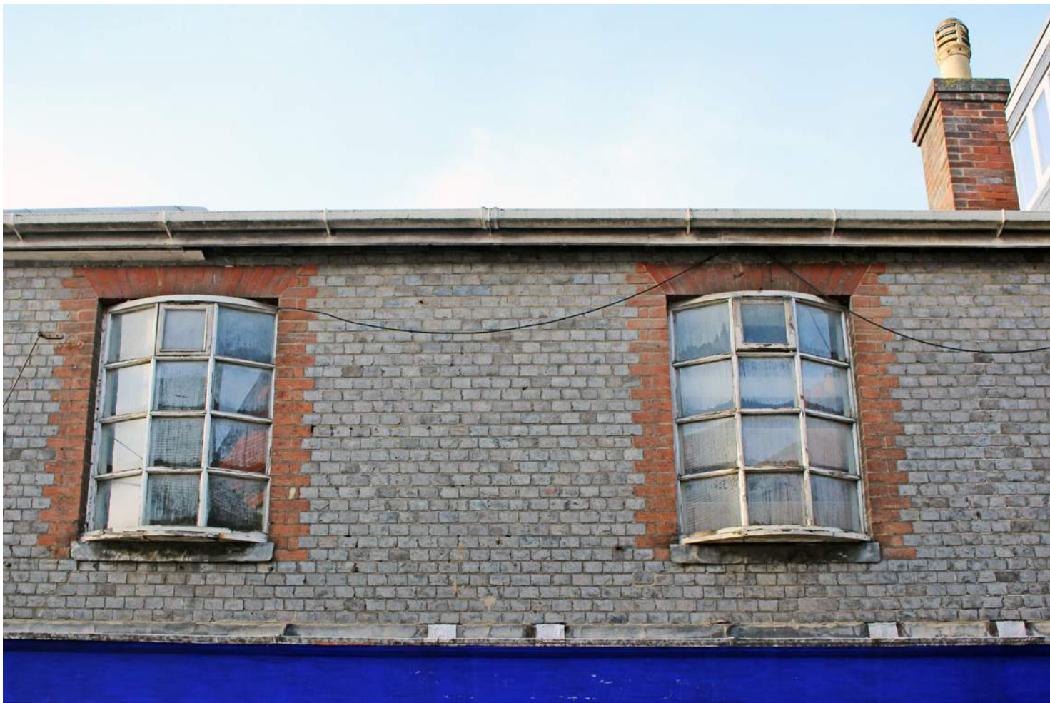
Figure 151: Non-original timber windows in disrepair
