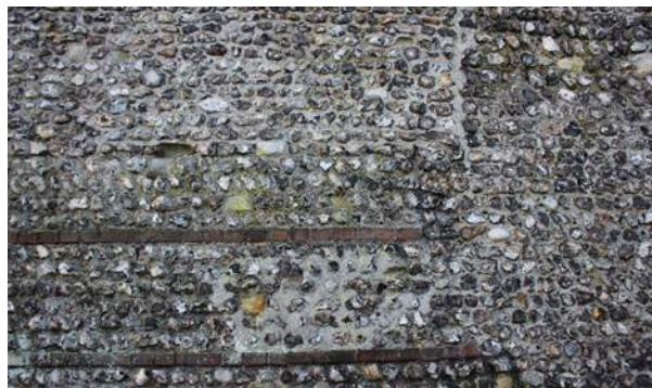
Figure 41: Flint boundary wall to Pelham House. The repair to the centre of the picture demonstrates the importance of consistency in pointing, the repair covering more of the flints in mortar
