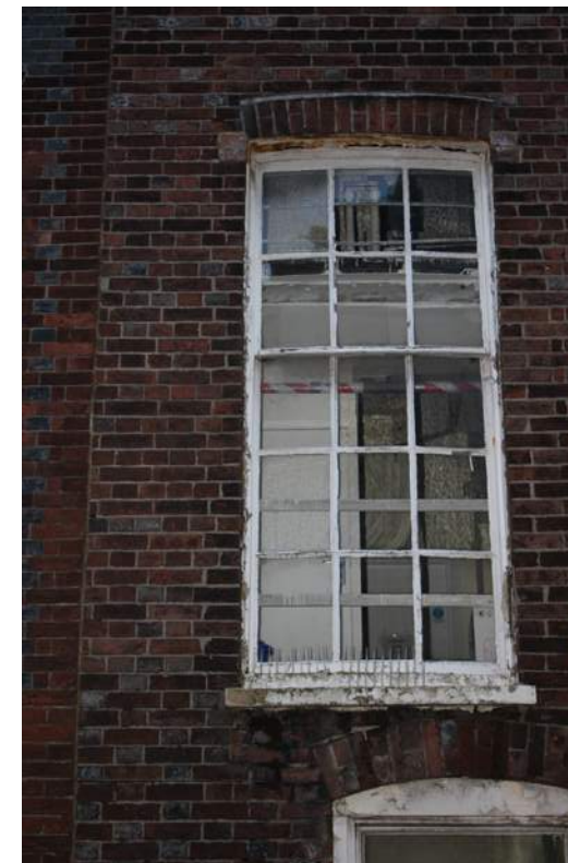
Figure 193: Pigeon spikes to the cill of a timber window in poor repair
