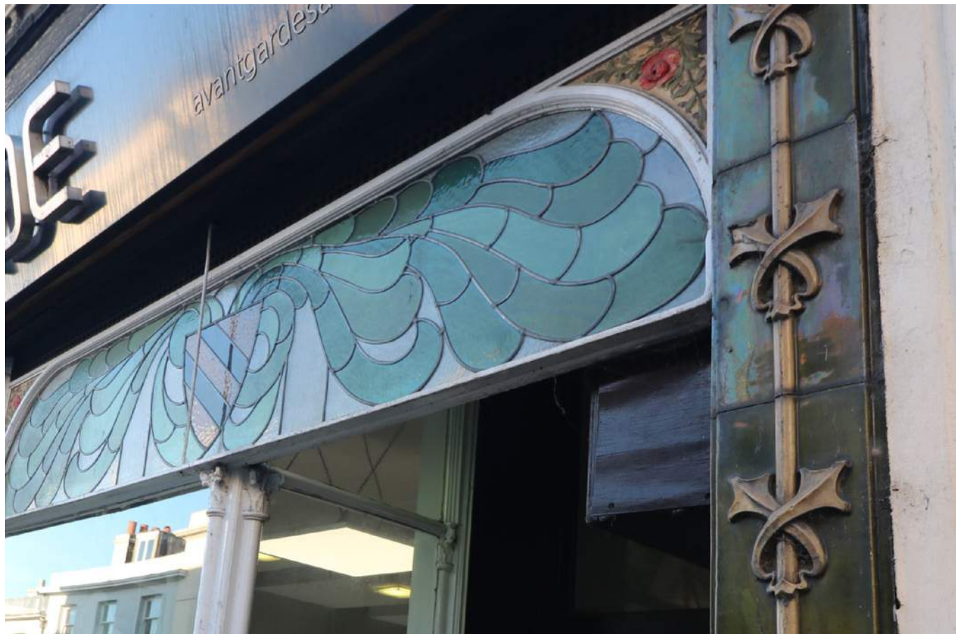
Figure 83: High Street shop front with slender transoms, a stained glass overlight and Late Victorian or Edwardian green glazed tiles to the edge of the shopfront
