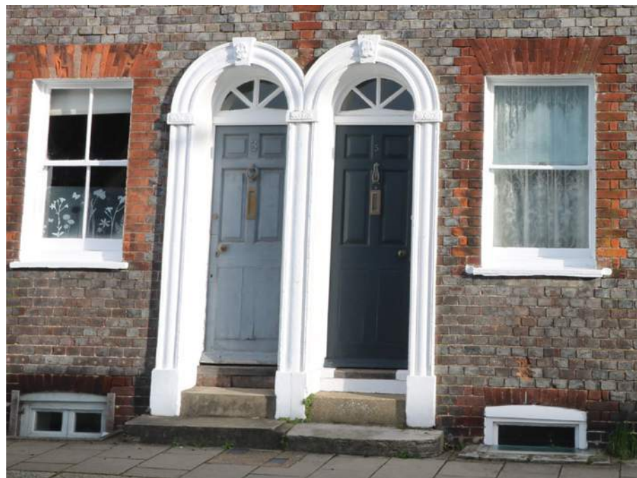
Figure 63: Highly articulated openings to a pairs of houses in Cliffe, thanks to the red brick window surround and moulded door surround
