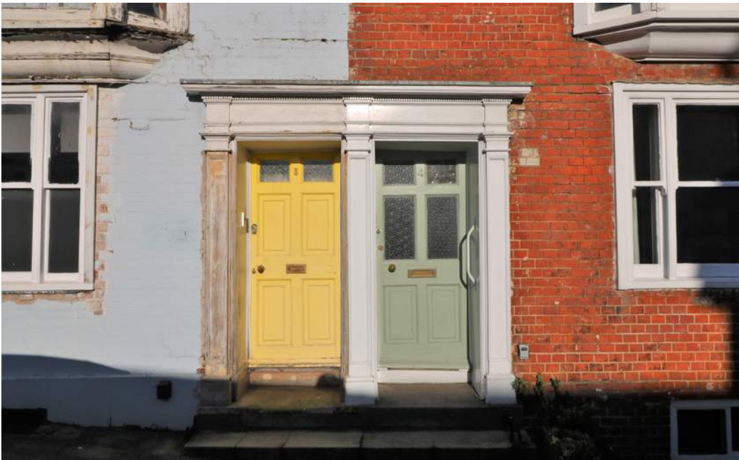
Figure 194: Neighbouring poorly-maintained and well-maintained houses, showing the impact of a lack of regular painting and maintenance on timberwork
