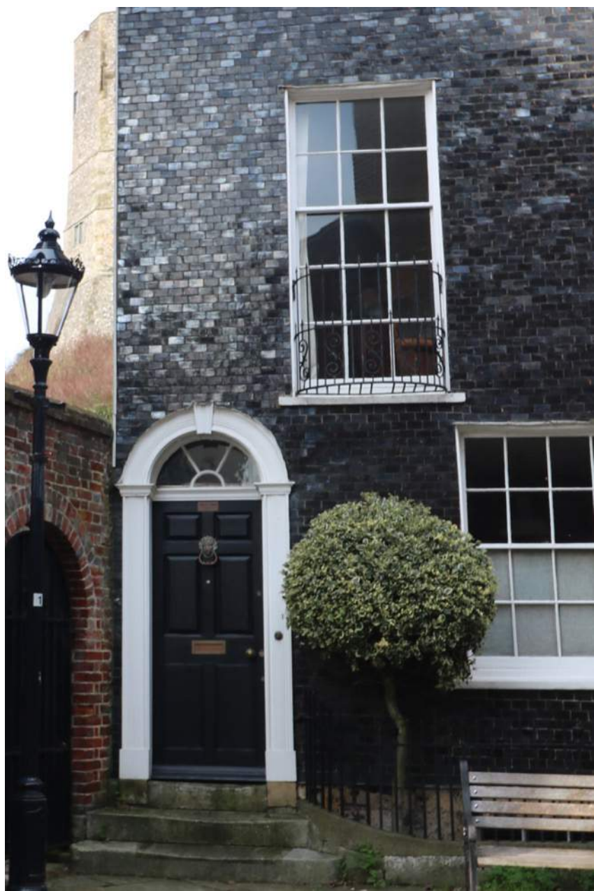
Figure 51: Vitrified mathematical tile to the façade of Bartholomew House. Note the lack of lintels over the openings
