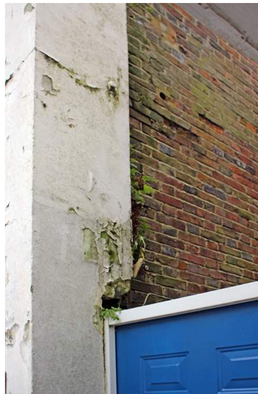
Figure 192: Building fabric in poor repair showing damp and algae due to continued water exposure
