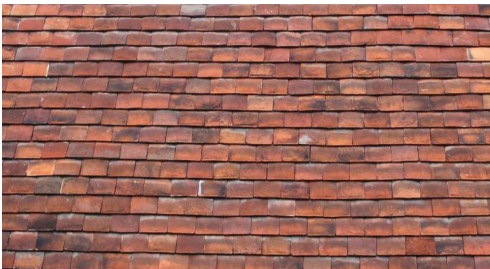
Figure 53: Handmade clay tiles cladding a wall surface . Clear variety in shape, colour and texture
