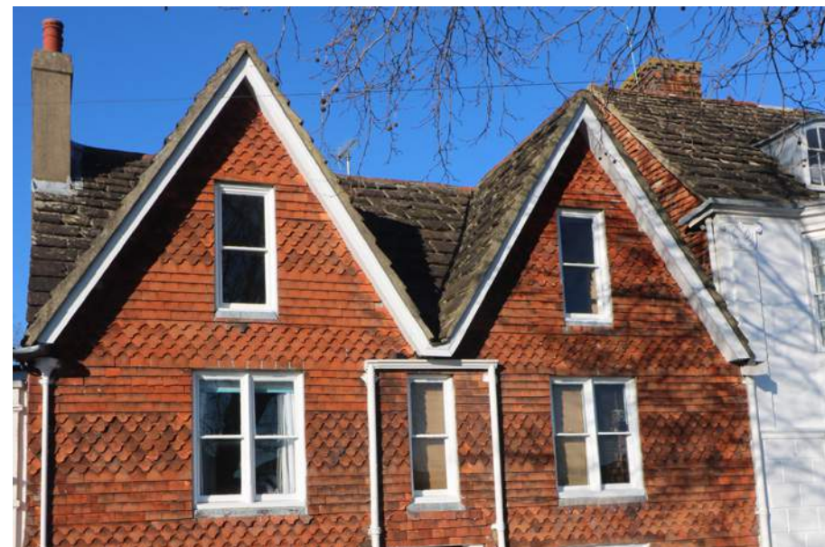
Figure 59: Horsham Stone slate roofs to Nos.55 and 56 Southover High Street. A steeper pitch is required than for slate
