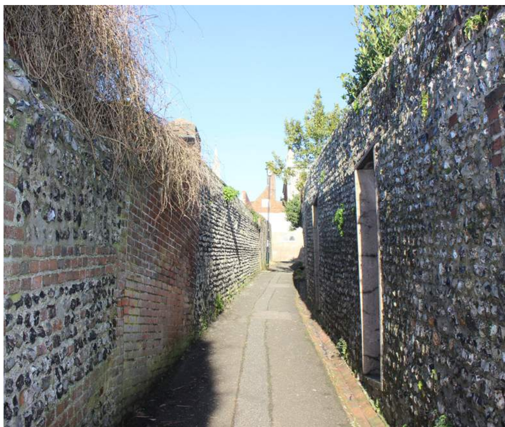
Figure 42: View along Paine's twitten. The flints protrude slightly beyond the surface of the pointing, creating a strong sense of texture
