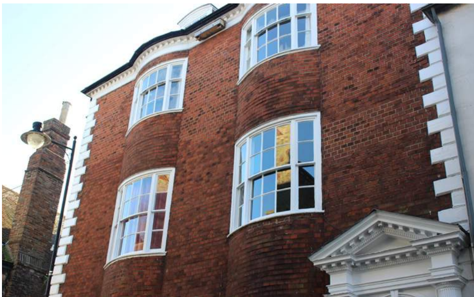
Figure 52: Mathematical tiles to Westgate House on the High Street. The large quoins have been added to obscure the end of the tiles and have no structural function. The junction between the bows and flat wall surface shows the join between the different sections of tile
