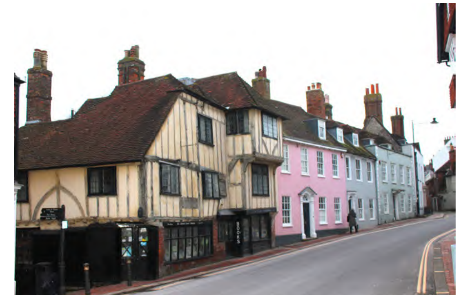
Figure 13: View along the High Street, illustrating changing architectural tastes, the jettied timber framed Fifteenth Century Bookshop adjacent to Georgian buildings. No.103 to the right of the picture is one of many medieval, timber-framed buildings in Lewes which has been retained behind a later, Georgian façade.
