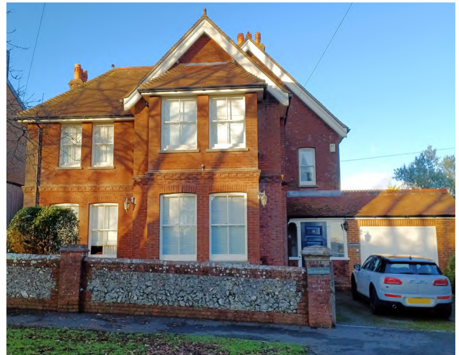
Figure 175: Typical brick and flint front boundary treatment
