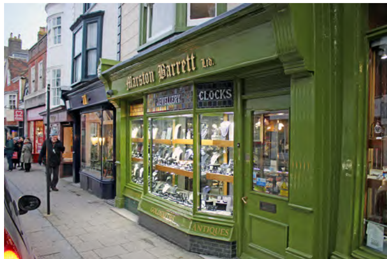
Figure 79: Marston Barrett’s particularly well preserved, late Victorian shopfront, which consists of a tiled stall-riser and retained stained glass, pilasters, consoles and fascia
