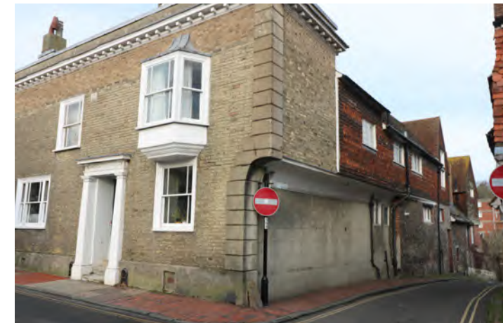
Figure 35: Jettied side return to Fairhall in Southover. The building dates to the 16th century, with a later brick front elevation
