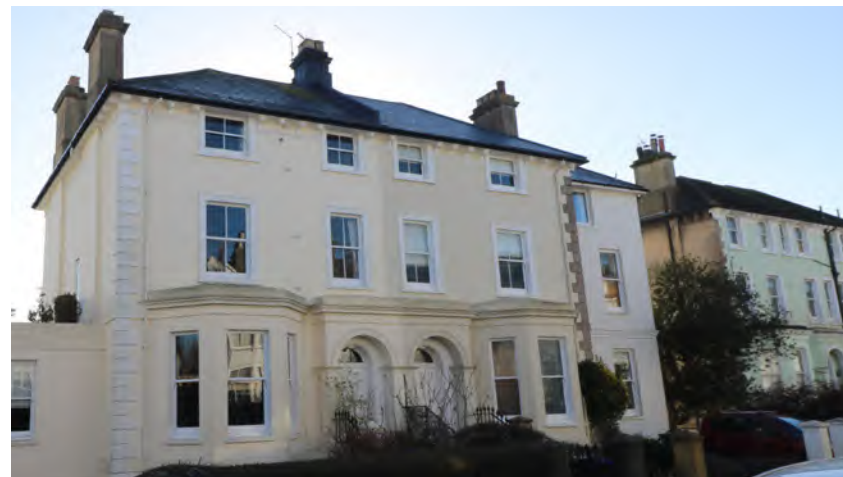
Figure 67: Stuccoed villas to St Anne’s Crescent, with shallow, arched porches, corbelled eaves, and quoins
