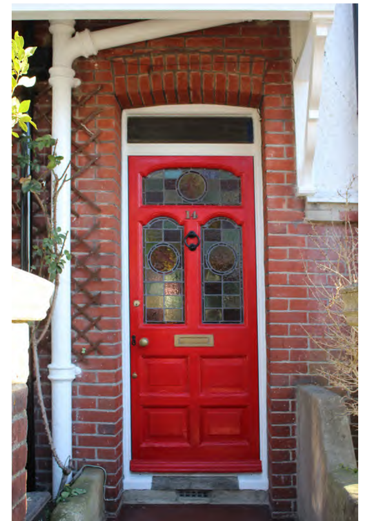
Figure 201: Historic door on St Swithun's Terrace with stained glass panels and modern replacement fanlight
