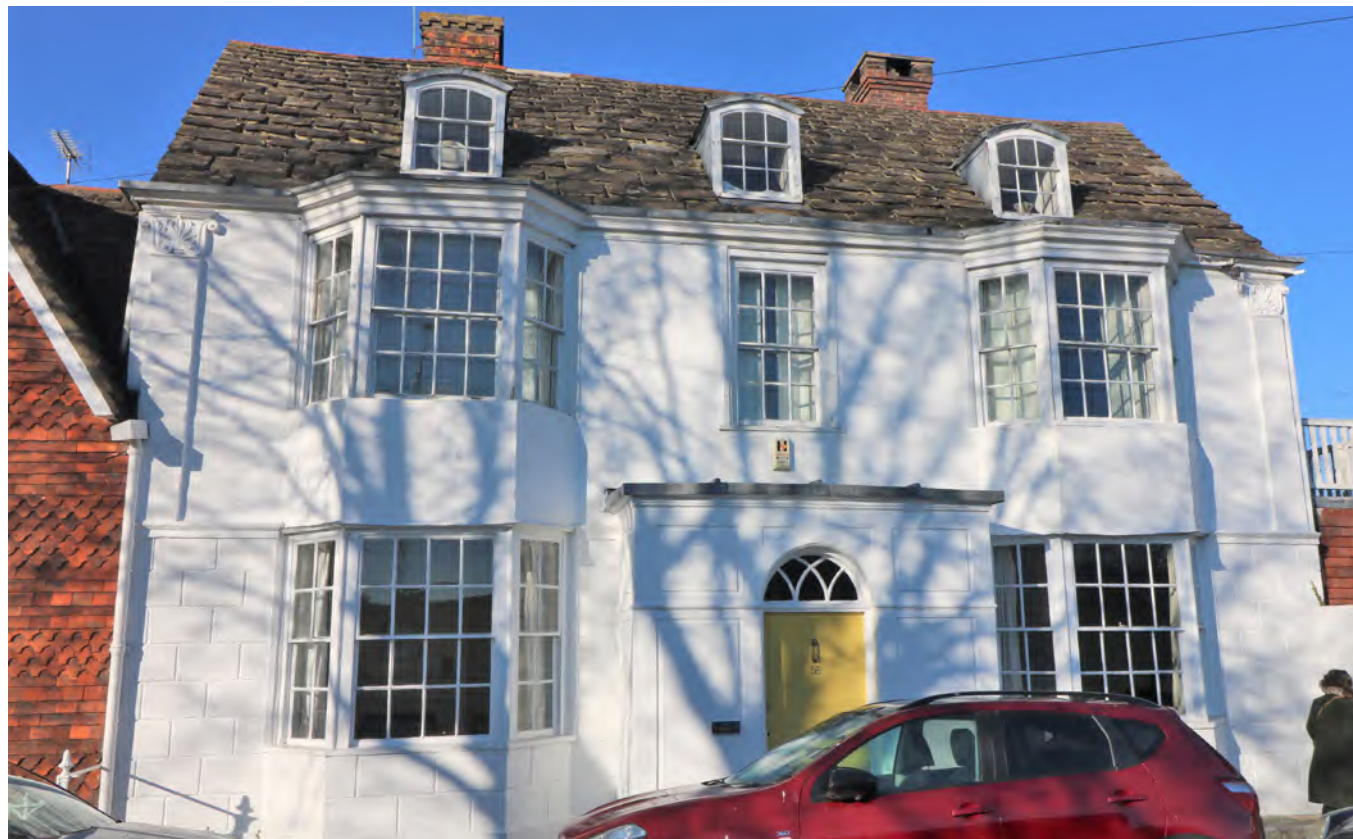
Figure 199: Finely detailed and proportioned historic doorway and windows
