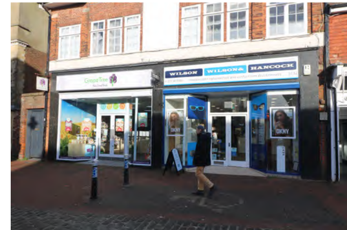
Figure 213: Unsympathetic modern shopfront and fascia signage to the High Street
