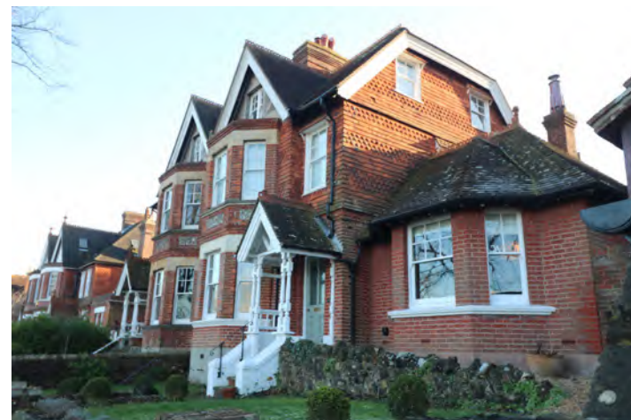
Figure 06: Villas on King Henry's Road
