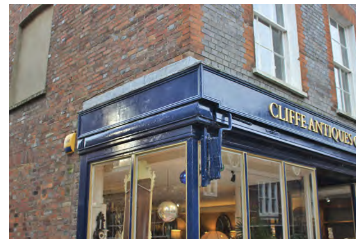
Figure 218: Historic ironwork intended to support a canopy on Cliffe High Street
