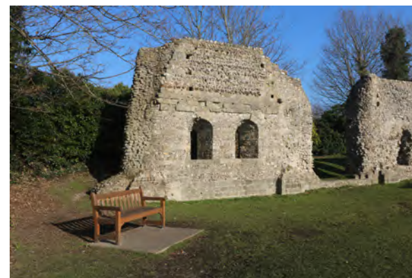
Figure 40: The use of flint in the Priory's walls is shown where the facing stone has been removed
