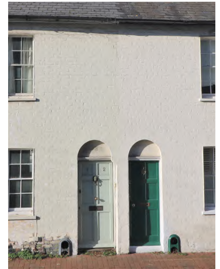
Figure 102: A pair of bootscrapers surviving in two 19th century terraces on Abinger Place
