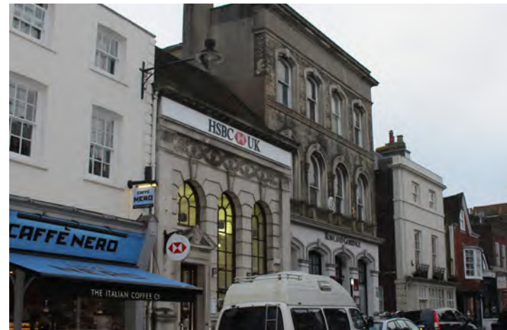
Figure 31: Nos.63 and 64 Lewes High Street – the former HSBC and Rowland Gorrings' office
