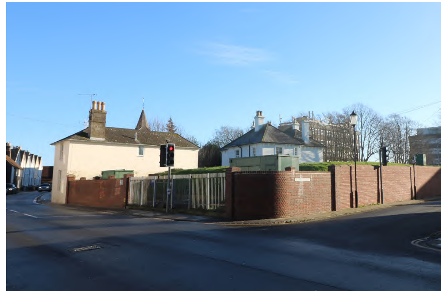
Figure 160: Covered reservoir to Western Road which features insufficient screening
