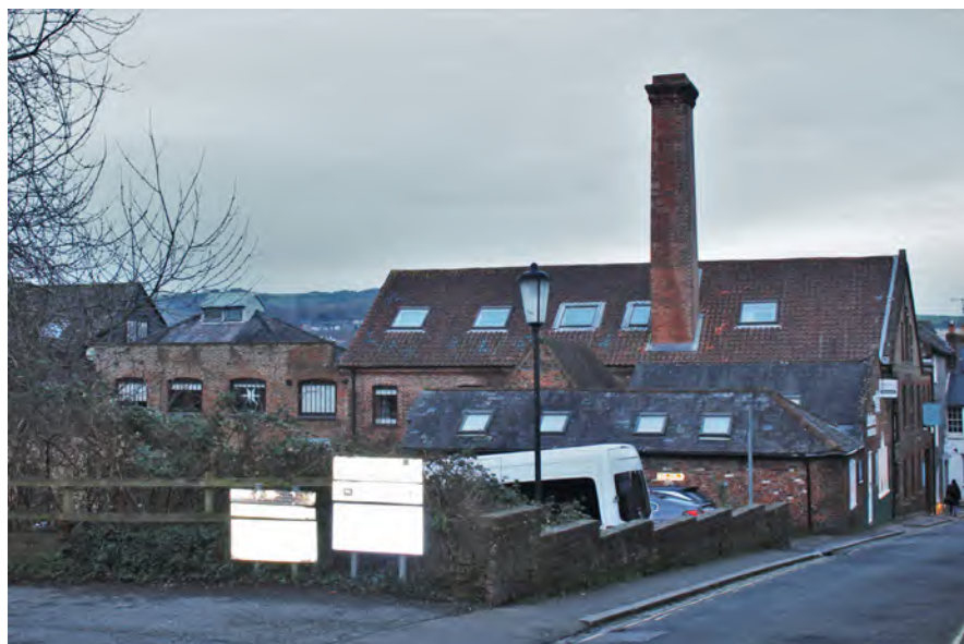
Figure 85: The former Broad's Candle Factory of the mid 19th century (now Old Needlemakers) viewed along Market Lane. The chimney is a prominent feature
