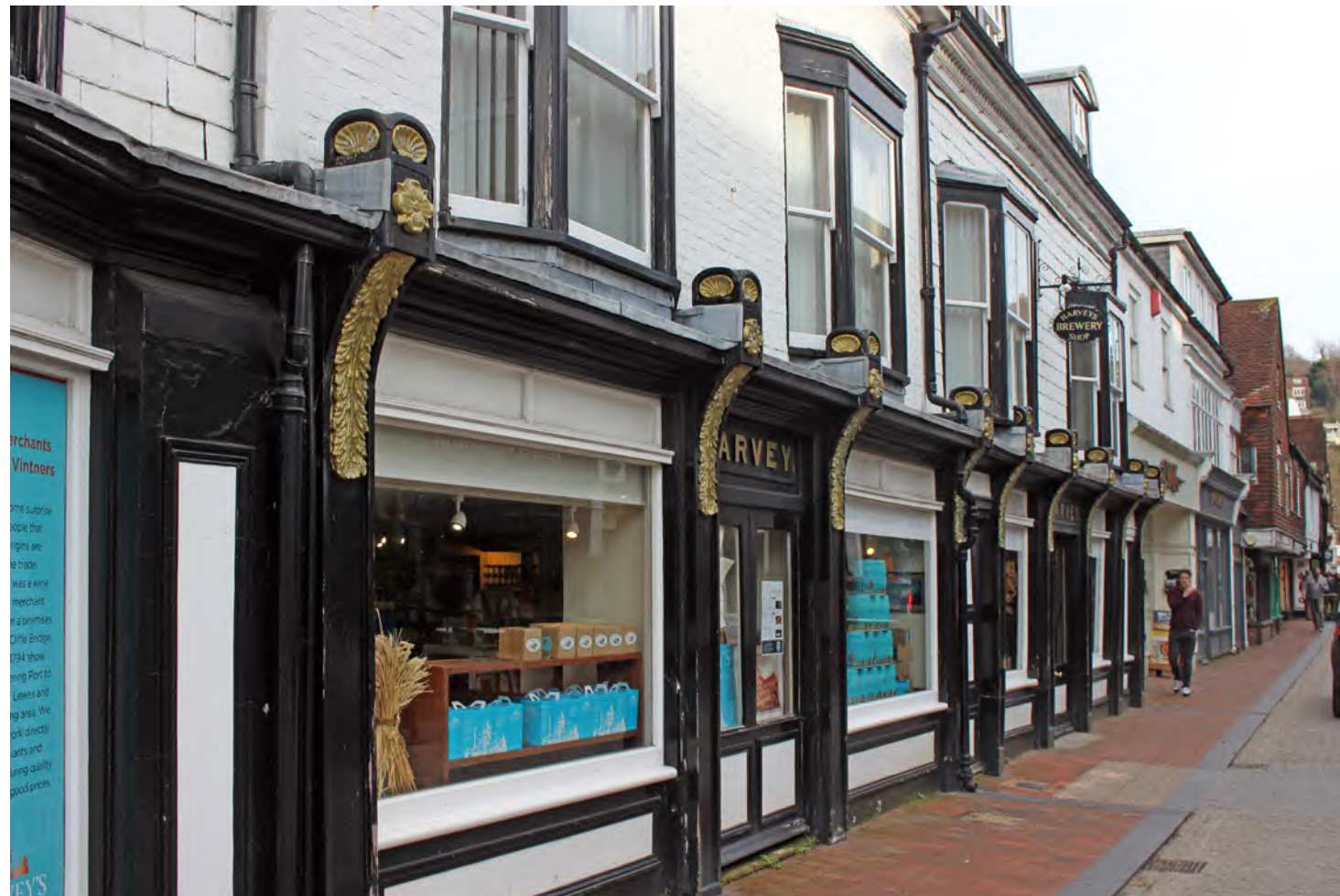
Figure 126: High-quality surviving shopfronts at Harvey's Brewery
