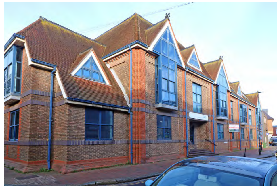
Figure 209: NHS building to Friars' Walk
