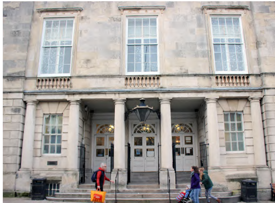
Figure 75: Classical detailing to the Crown Court façade , designed by John Johnson and completed in 1812
