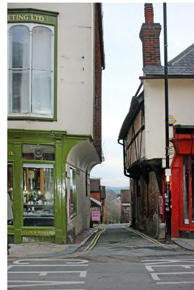
Figure 146: Jettied timber frame buildings to the north end of St Martin’s Lane
