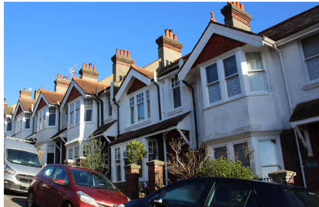
Figure 55: Roughcast render façades to St Swithun’s Terrace
