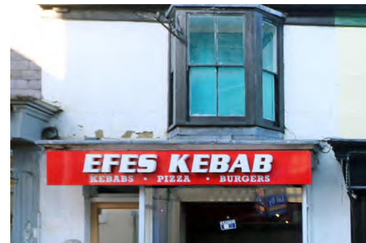
Figure 214: Poorly proportioned low-quality plastic signage
