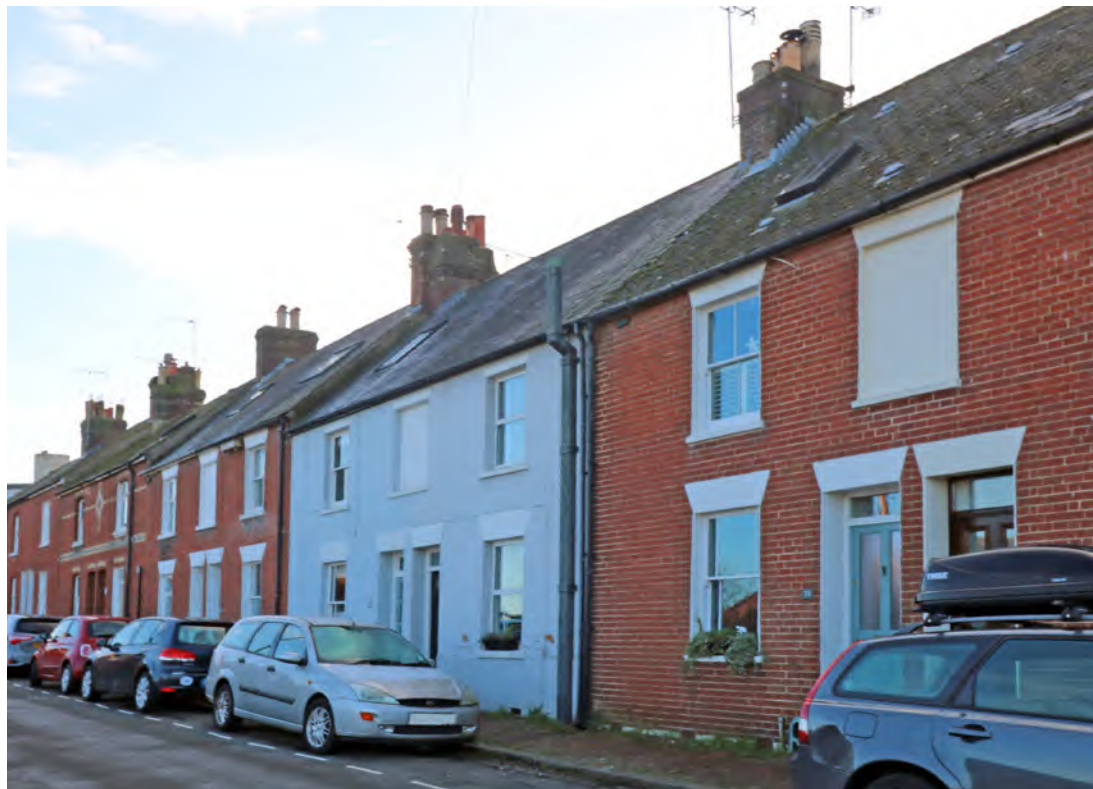
Figure 191: Bulky roof lights to Valence Road
