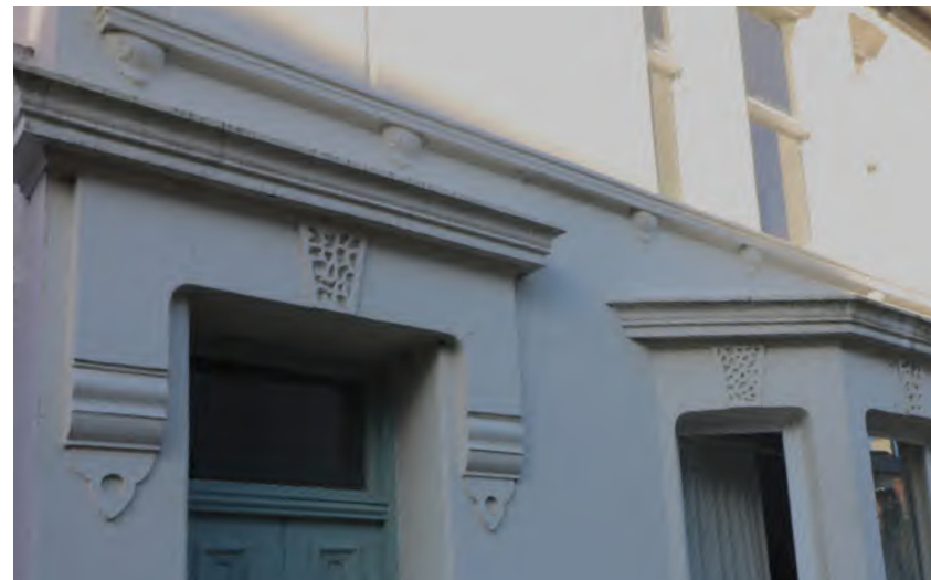
Figure 66: High-quality detailing to a terraced house in the Pells, including rusticated keystones, a corbelled door surround, and moulding to the cill of the first floor windows
