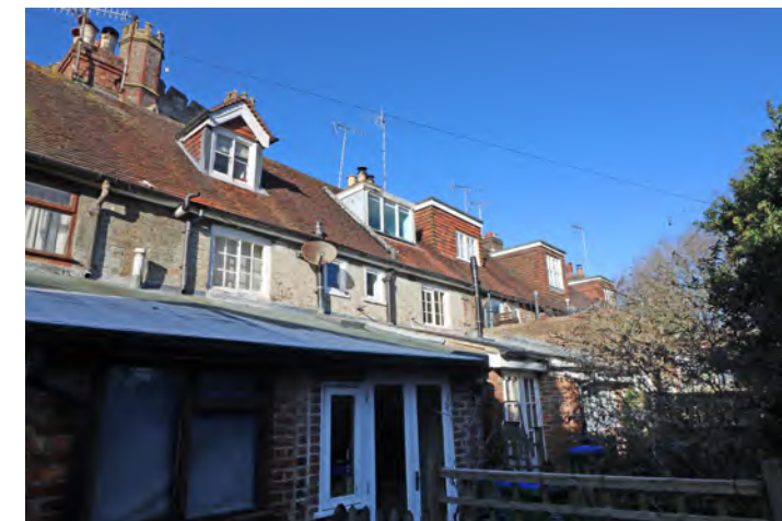
Figure 187: Cluttered roofscape to the rear of buildings along Church Row
