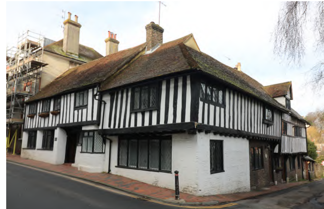
Figure 61: Timber-framed Nos.49-50 on Southover High Street, which dates to the 16th century. The building jetties to both the front and side return and has leaded casement windows.
