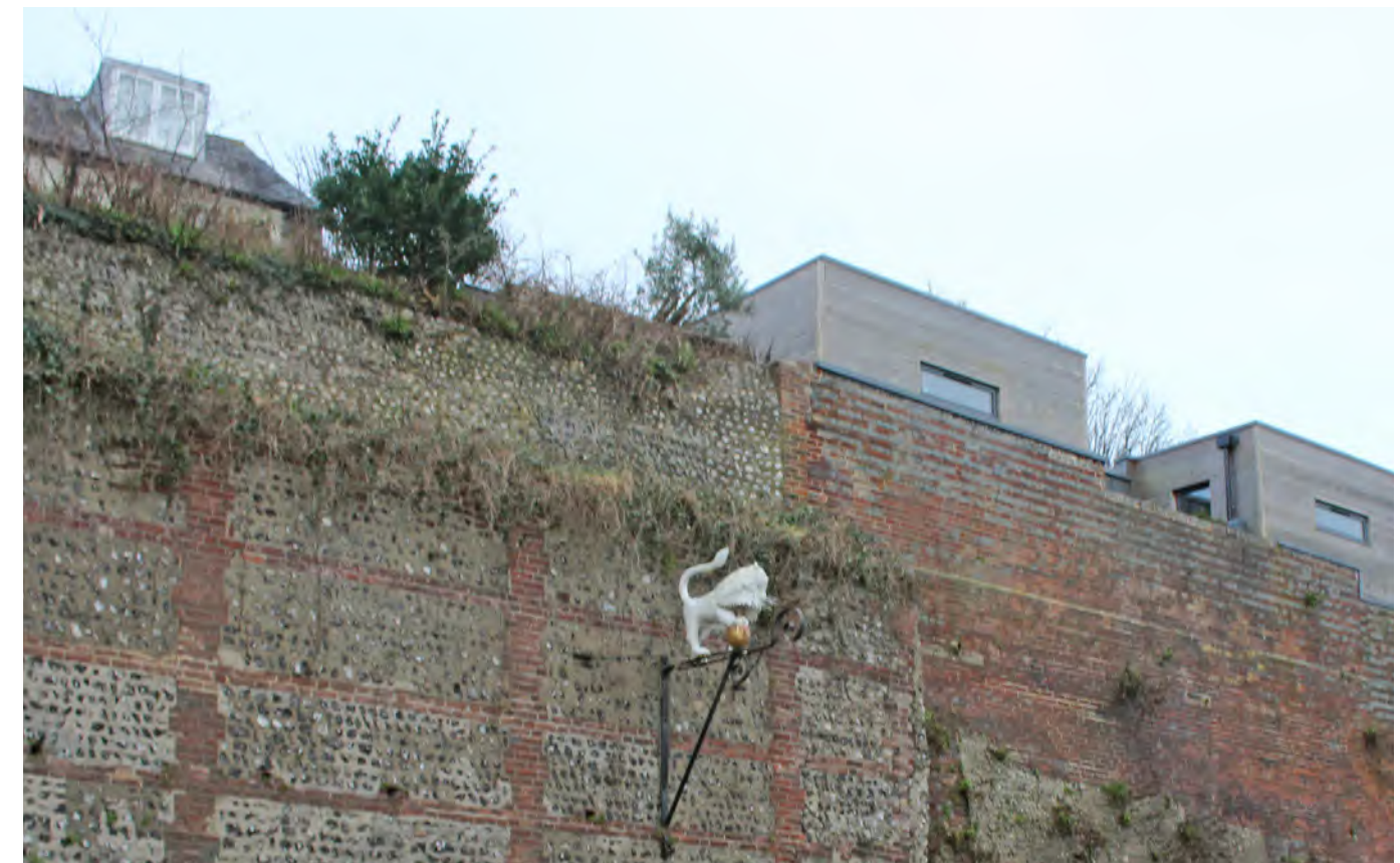
Figure 240: Remains of the town walls along Westgate Street, dating to the 13th or 14th centuries, with potential pre-Conquest foundations
