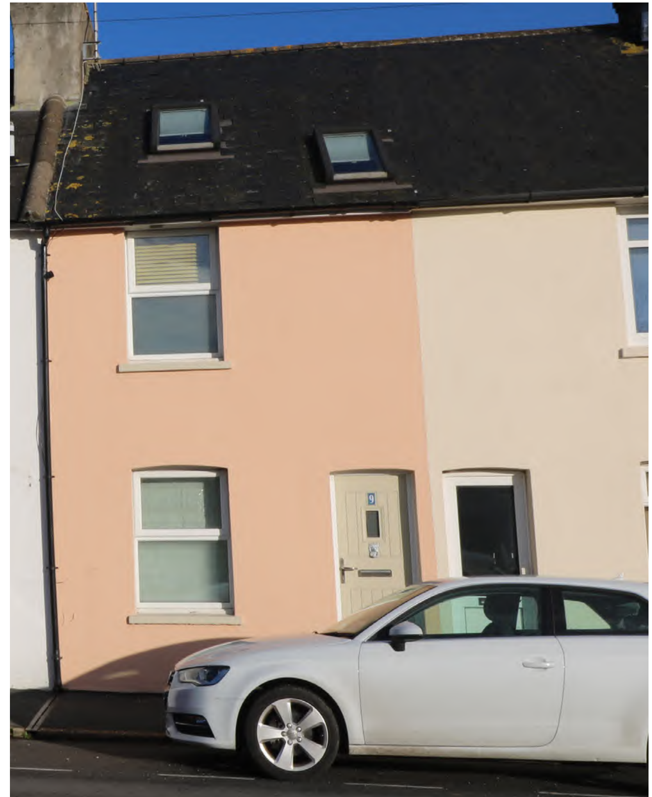
Figure 177: Visually intrusive, non-conservation skylights and detracting uPVC windows
