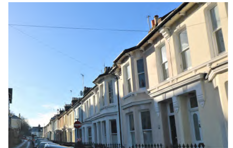
Figure 197: Visually prominent antennae located to the front pitch of roofs on tall poles
