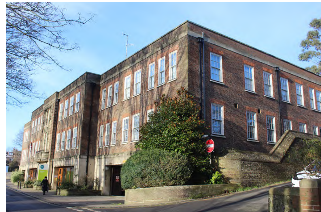
Figure 29: Southover House, formerly offices of Lewes and Eastbourne District Council
