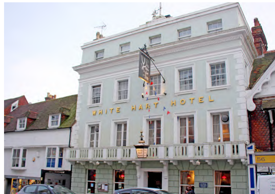
Figure 242: White Hart Hotel, a 16th century building refronted in a classical style in the 19th century
