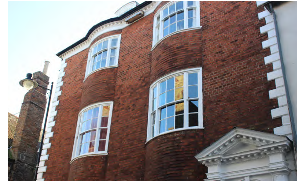
Figure 52: Mathematical tiles to Westgate House on the High Street. The large quoins have been added to obscure the end of the tiles and have no structural function. The junction between the bows and flat wall surface shows the join between the different sections of tile
