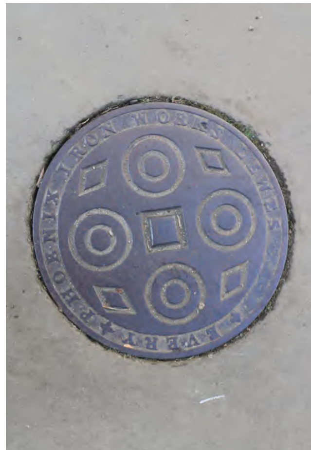
Figure 100: Coal hole cover from John Every’s Phoenix Ironworks in Lewes
