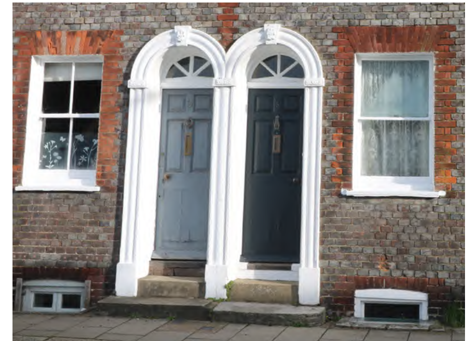
Figure 63: Highly articulated openings to a pairs of houses in Cliffe, thanks to the red brick window surround and moulded door surround
