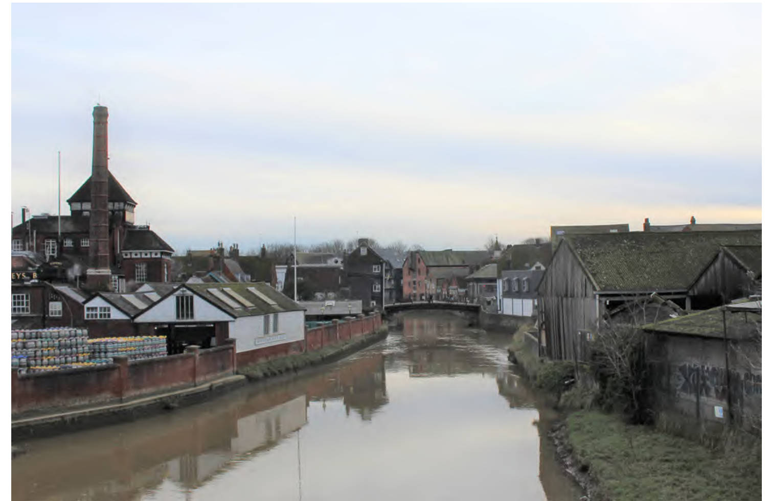
Figure 244: View towards Cliffe Bridge with the rear of Harvey’s Brewery visible to the left
