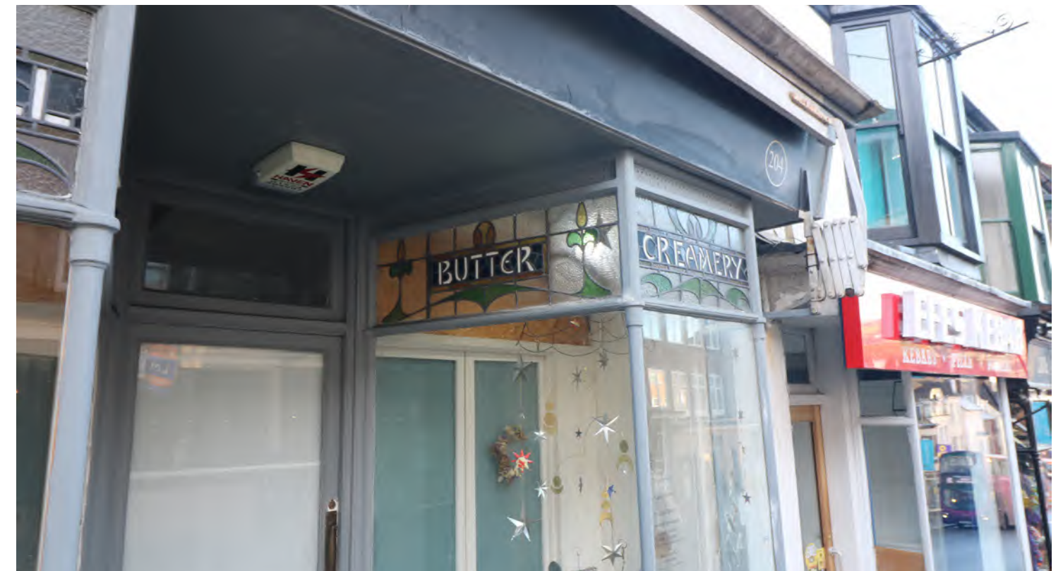
Figure 136: Stained glass overlight to 207 High Street
