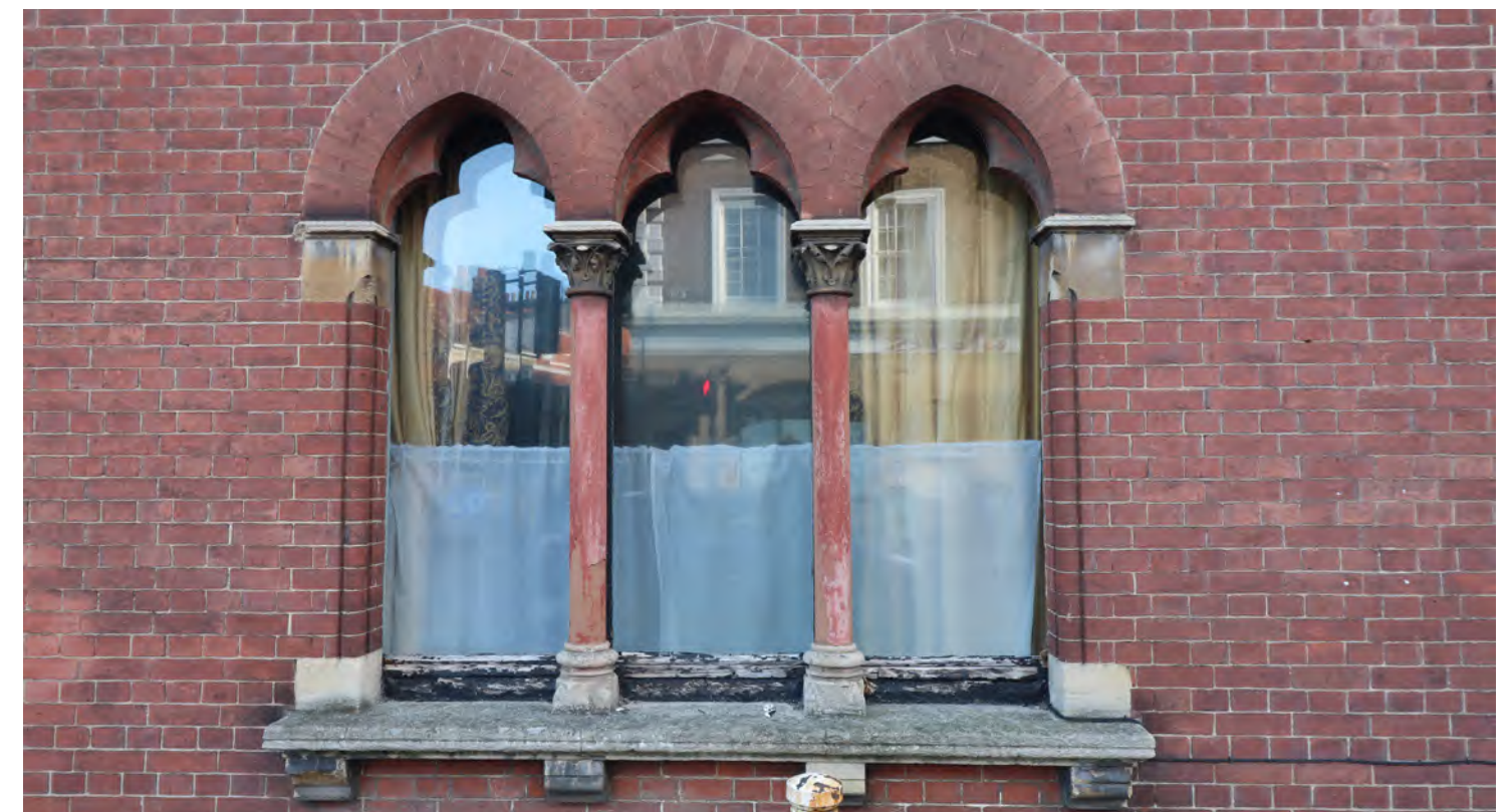
Figure 137: Trefoil windows to the Fitzroy Memorial Library
