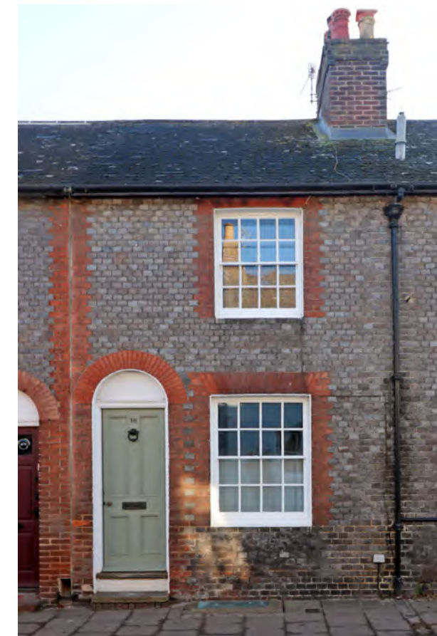
Figure 65: Polychromatic terrace to Priory Street
