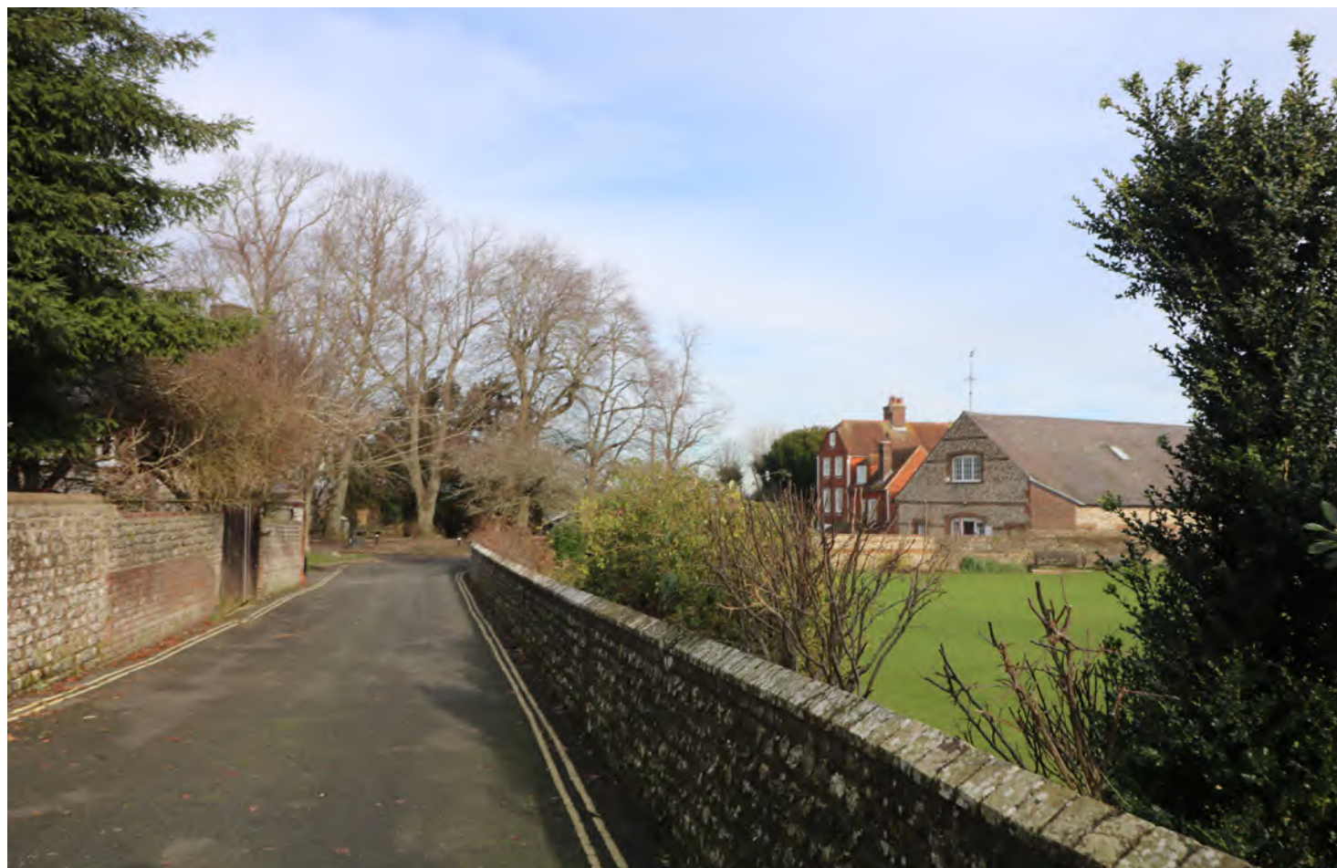
Figure 148: Flint boundary walls to the Castle Precinct
