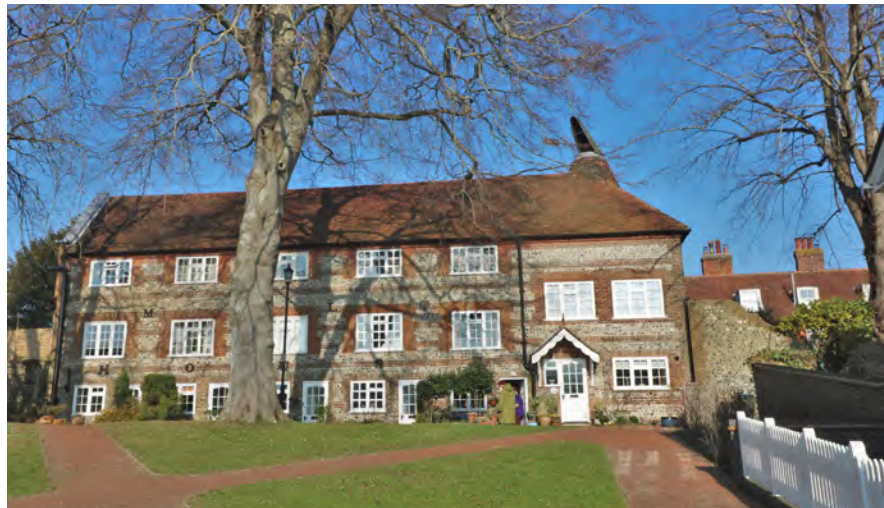
Figure 84: The former Verrall's malthouse in Southover, built in the mid 19th century. The roof cowl for drawing air into the kiln is visible to the right-hand hipped end.
