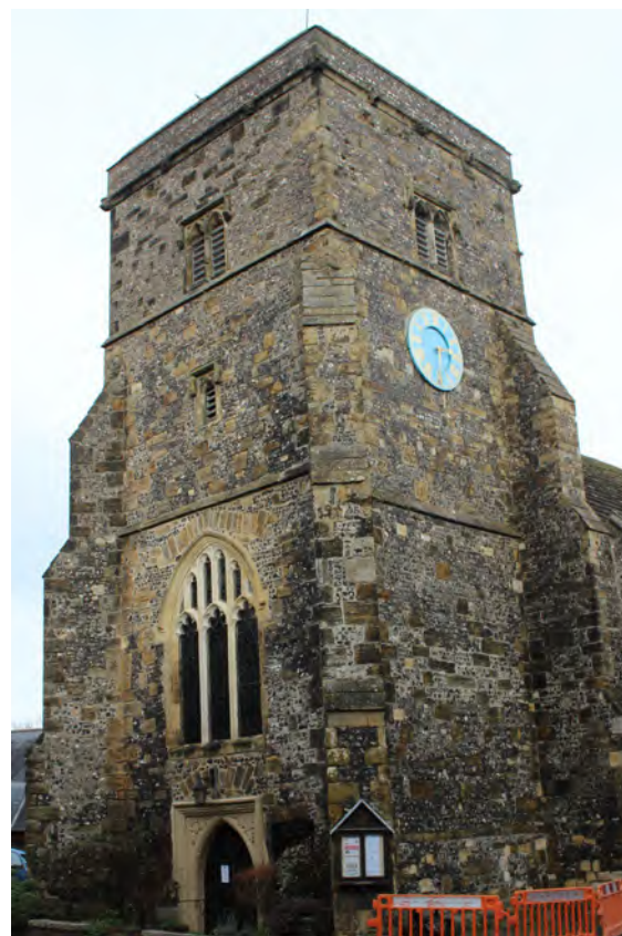
Figure 39: The tower of the church of St Thomas à Becket in Cliffe demonstrates how flint is not used at edges of wall surfaces, with stone introduced at the edges of the buttresses or joins where the buttresses meet the tower
