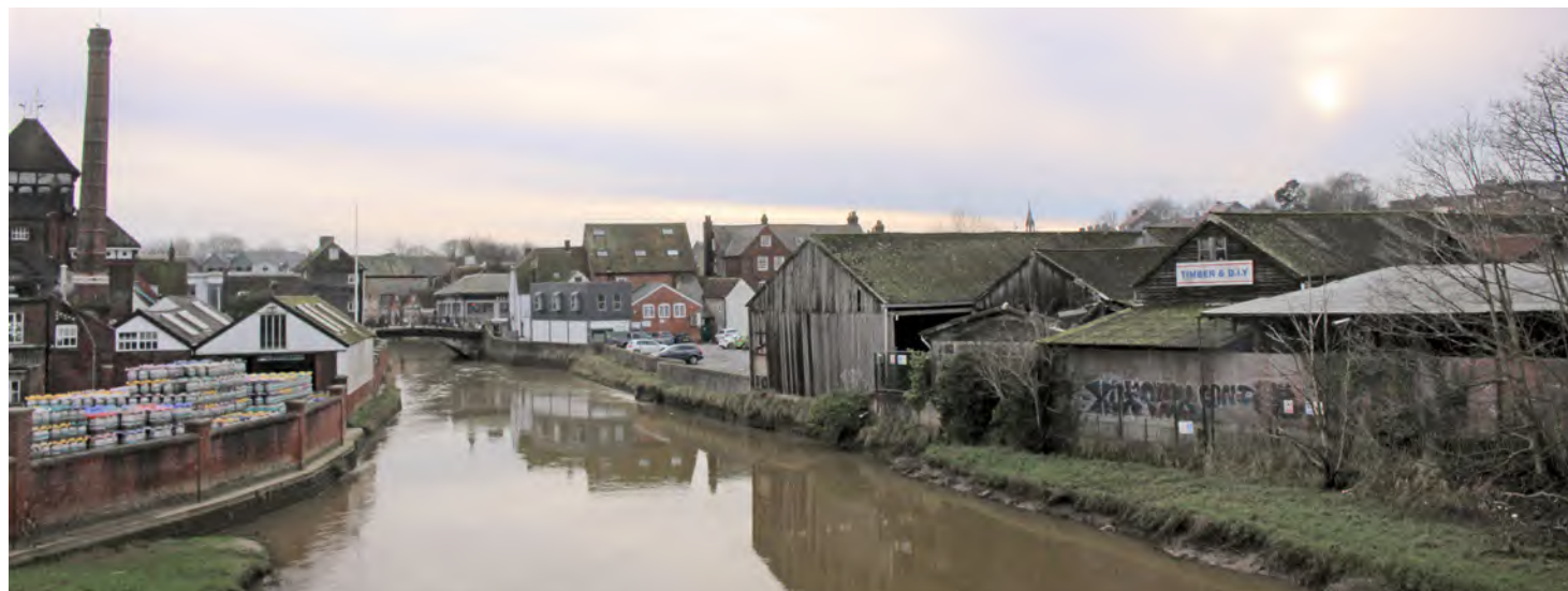
Figure 140: View from the Phoenix Causeway
