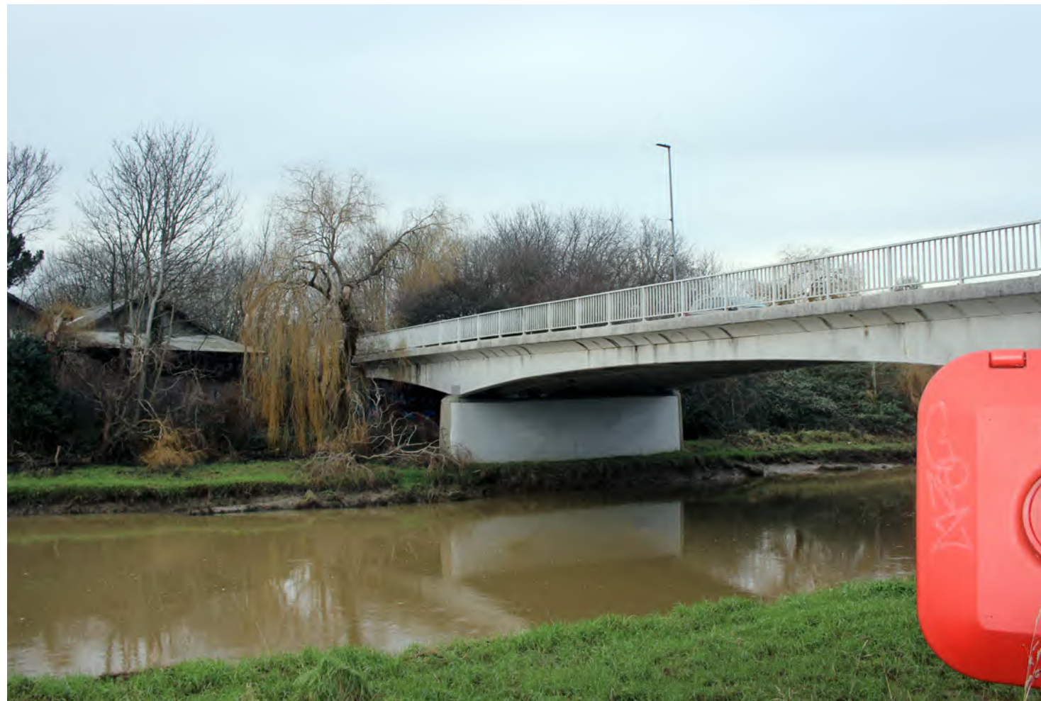
Figure 260: View of the Phoenix Causeway crossing the River Ouse
