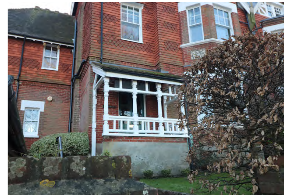
Figure 72: Highly articulated porch to a house on King Henry's Road in the Wallands. Note the change between brick at ground floor level and hung-tile to the upper floors, and small infill panel rubblestone to the bay window.
