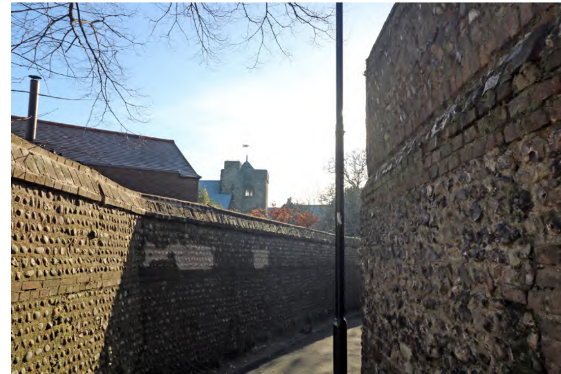
Figure 132: Church Twitten enclosed by flint and brick walls, which are a distinctive feature of the town, reinforcing the street pattern established in the Anglo-Saxon period
