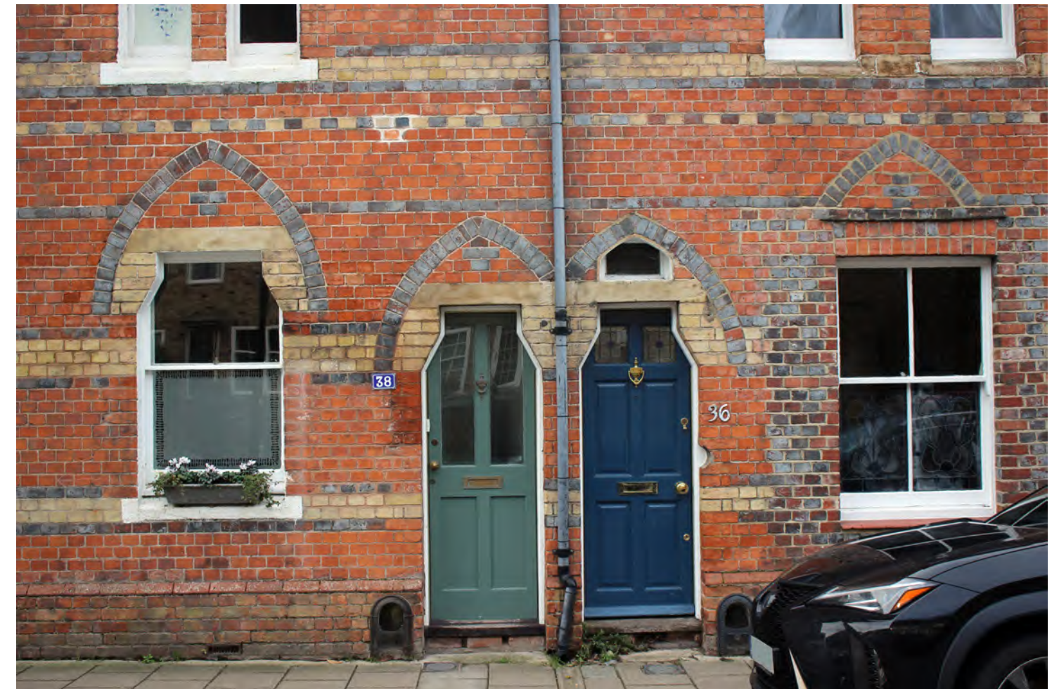
Figure 127: Characterful houses to South Street with brick polychromy reflecting pointed Gothic arches
