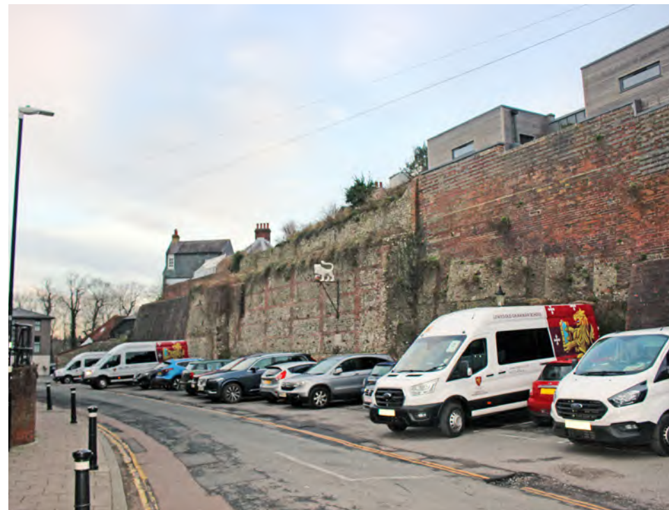
Figure 234: Prominent parking and poor quality road surfacing to Westgate Street
