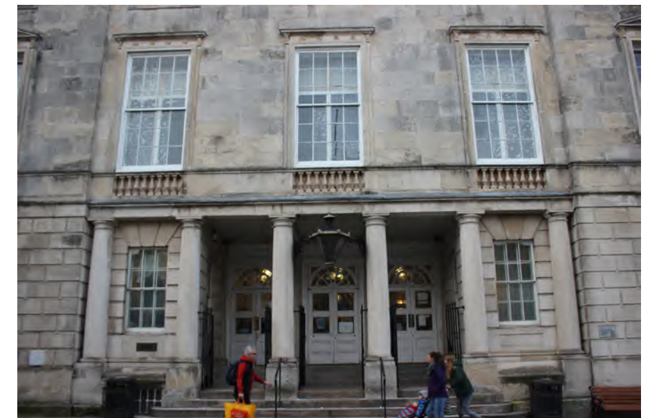
Figure 44: Ashlar Portland Stone used at Lewes Crown Court (former the County Hall)
