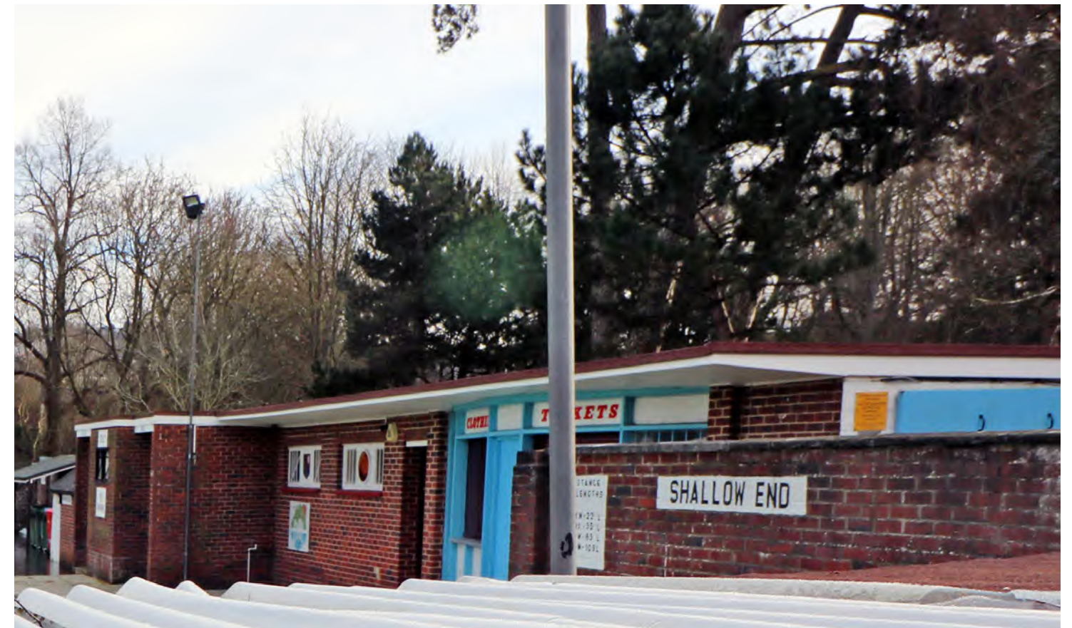
Figure 162: Ancillary buildings at the Pells Pool
