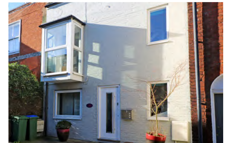
Figure 188: Unsympathetic uPVC windows to St John Street
