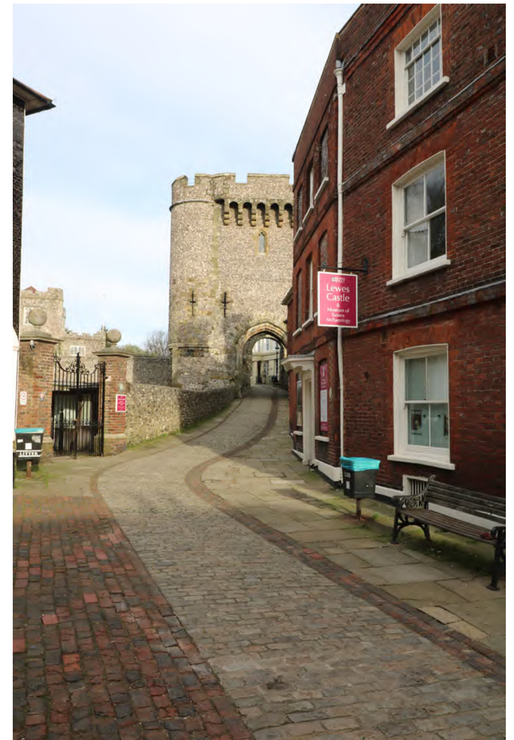
Figure 98: Modern stone setts have been reinstated adjacent to historic brick and York Stone pavers on Castle Gate. The now removed tarmac finish was an alien intrusion in a sensitive historic context
