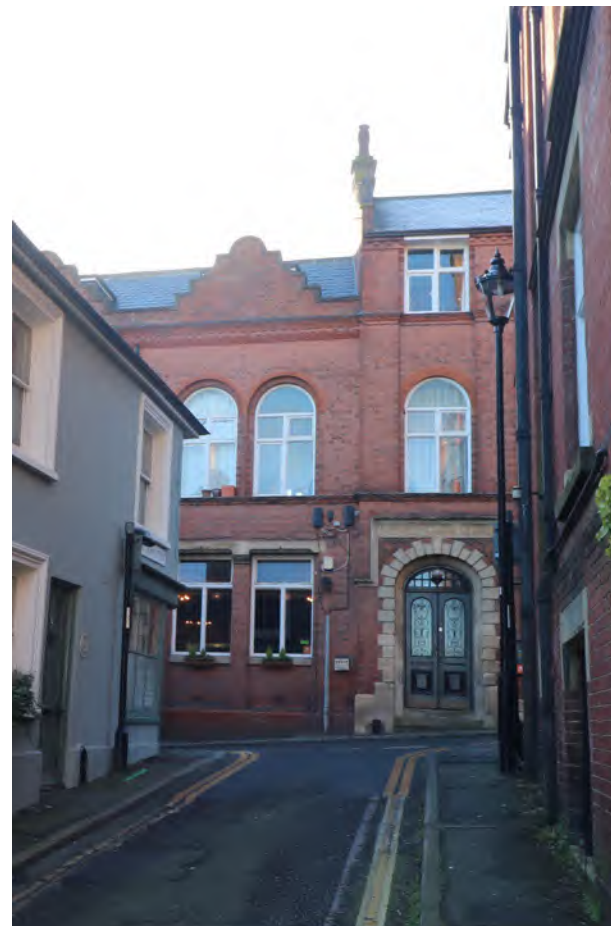
Figure 45: Stone door surround to No.18 East Street, with the stone window lintels to the Old Police Station visible to the right
