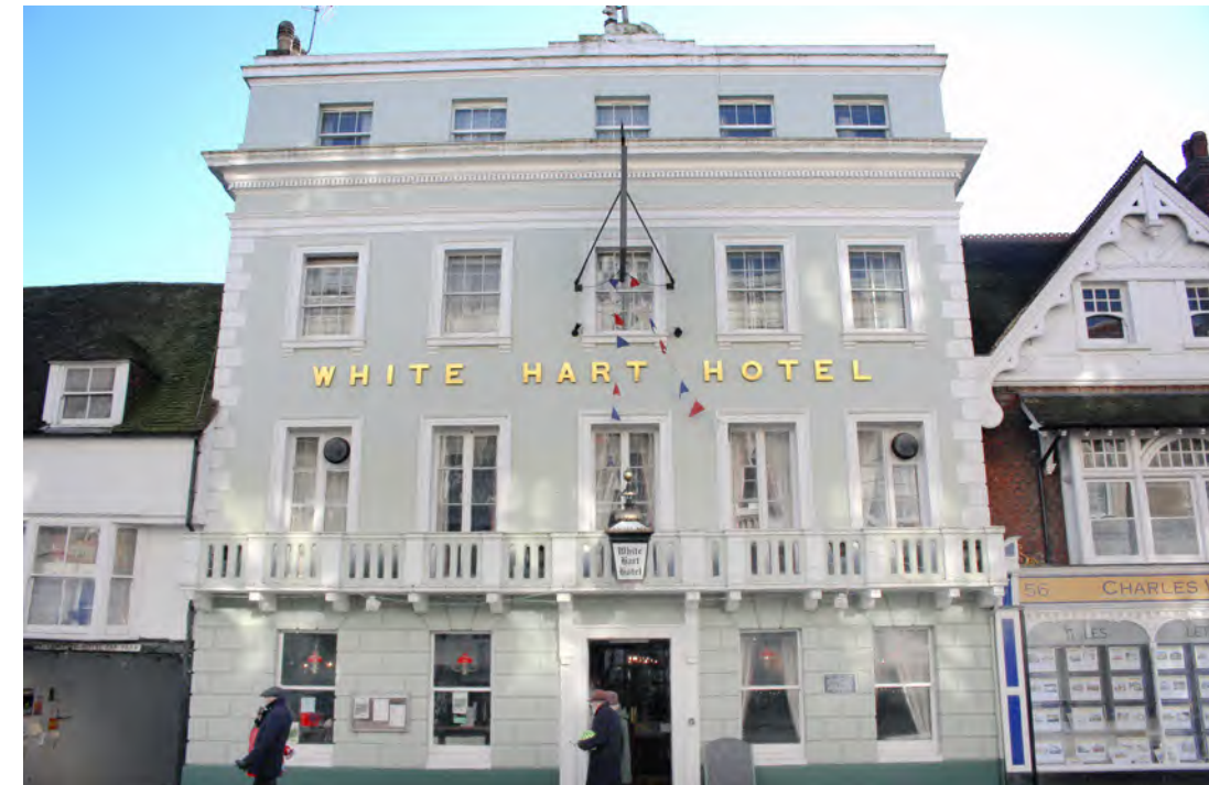
Figure 60: Classical façade to the White Hart Hotel, a mid 19th century refronting of a medieval building
