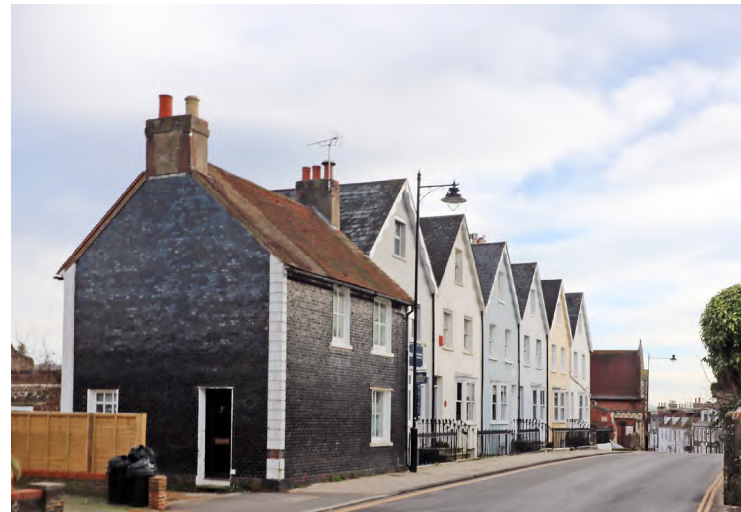
Figure 153: View looking east along the curving High Street
