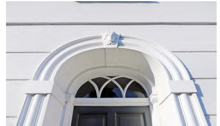
Figure 69: Regency door surround and fanlight in Southover
