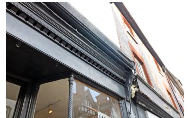
Figure 216: Well-detailed shopfront on the High Street with historic canopy ironwork
