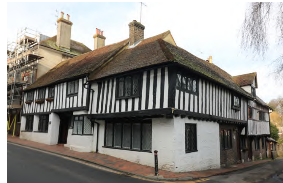
Figure 182: Historic timber-framing at 49-50 Southover High Street
