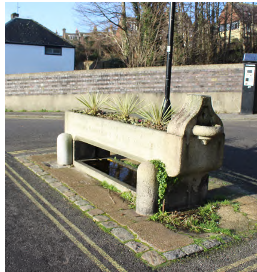
Figure 101: Former cattle trough to the south end of Watergate Lane
