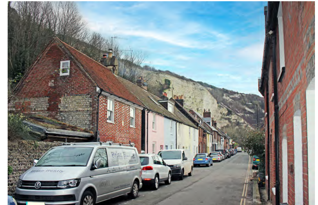
Figure 110: View along South Street showing the fine-grained terraces along the street and the chalk cliff rearing behind the Cliffe character area
