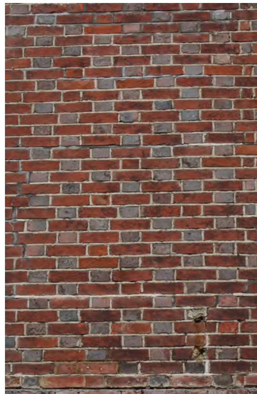
Figure 48: Grey headers and red stretchers laid in Flemish bond
