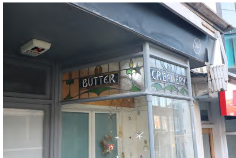
Figure 81: Detail of the shopfront of No.205 Lewes High Street, formerly a creamery, showing the stained glass overlight, canopy brackets and slender transoms
