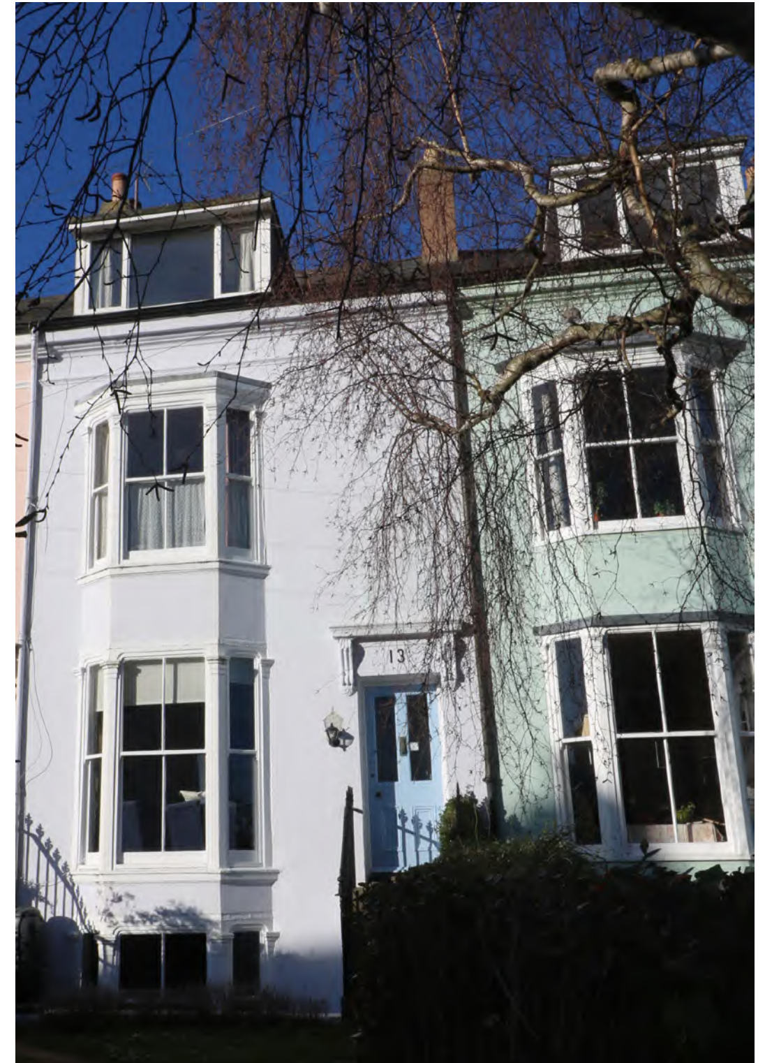
Figure 56: Stuccoed terrace on St Anne’s Crescent
