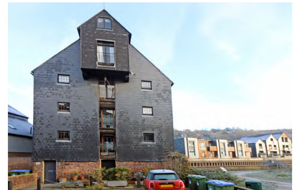
Figure 210: A refurbished wharf building with recent housing developments over the Ouse in Cliffe in the background
