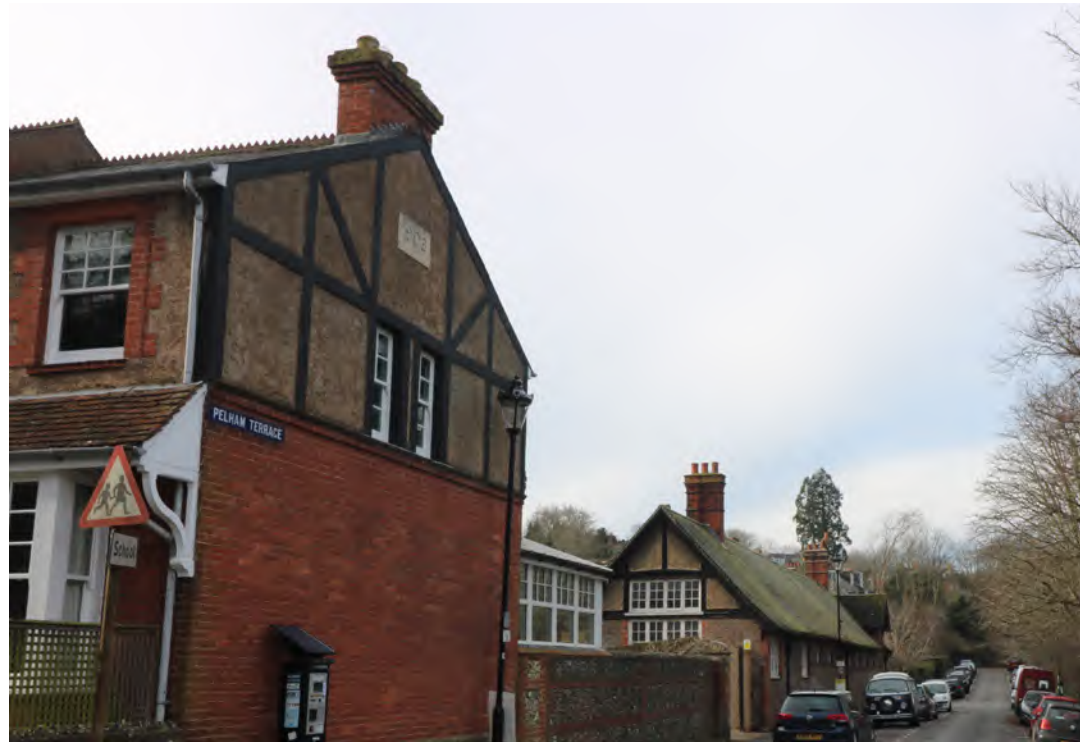
Figure 54: Roughcast render side returns of the former Pells School and end of the terrace to St John’s Hill
