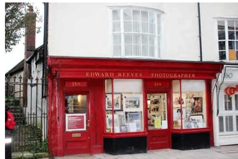
Figure 80: Edward Reeves’s 19th century shopfront, which retains a stall-riser, recessed entrance, fascia and canopy ironwork
