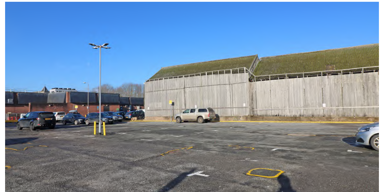
Figure 207: Eastgate Car Park and Eastgate Wharf
