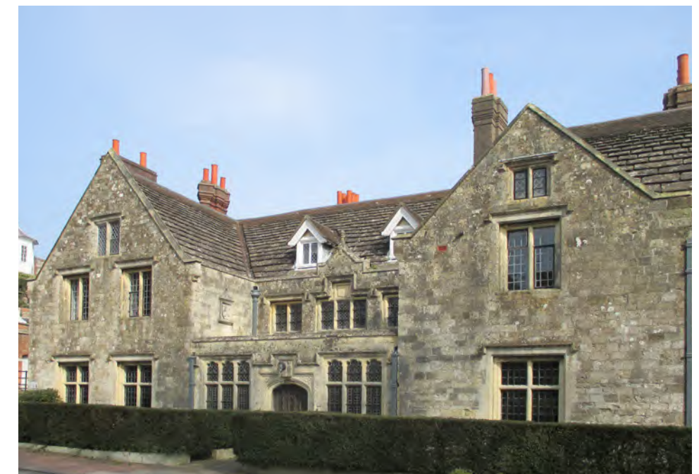
Figure 243: Southover Grange, built in the late 16th century with dressed Caen stone salvaged from the Priory (The Antiquary, Wikimedia (CC BY-SA 4.0))
