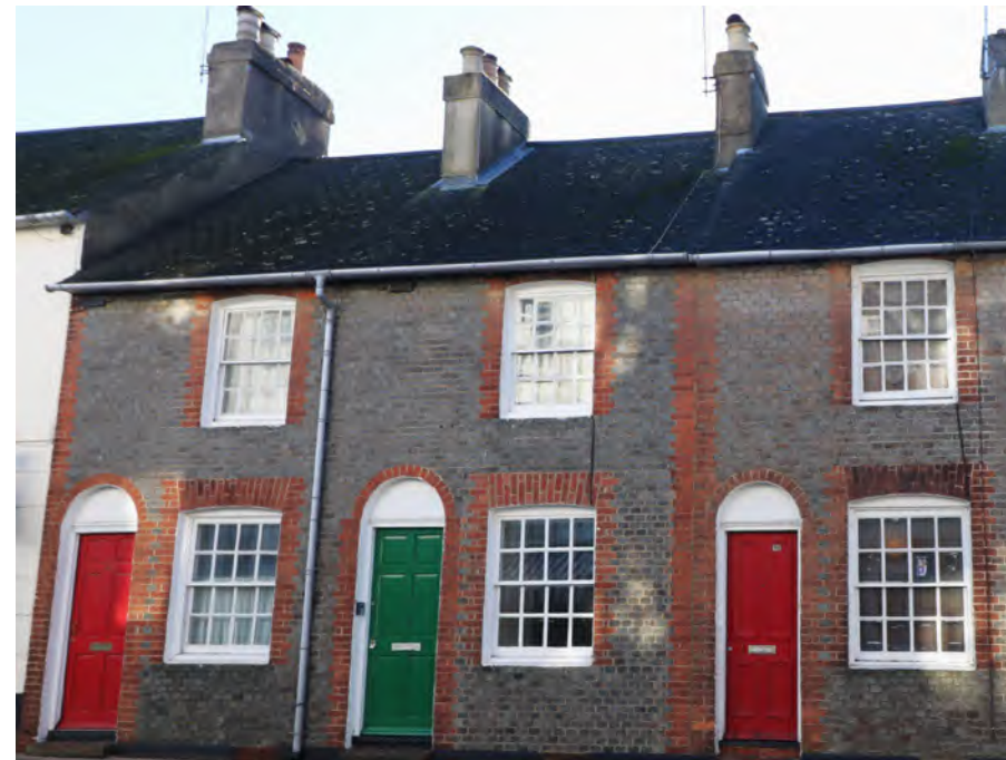
Figure 62: Polychromatic brick terrace on Western Road, with segmental arches, rather than flat ones.
