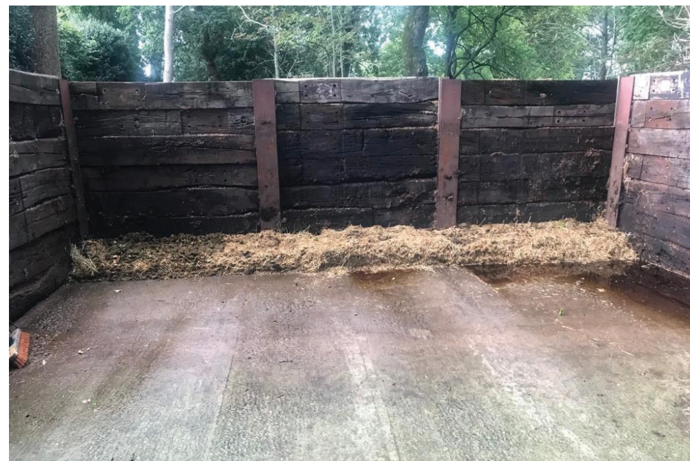
FIGURE 7: MUCK HEAP CONSTRUCTED WITH A NON-PERMEABLE BASE
