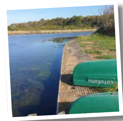
Further riverbank repairs for watersport access at SSCP © Buzz Active
