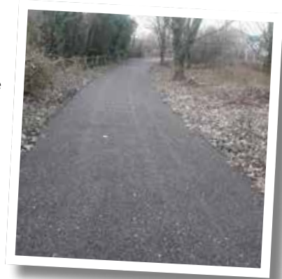
Completed Chilcomb route on SDW now bypassing busy A31 roundabout © SDNPA
