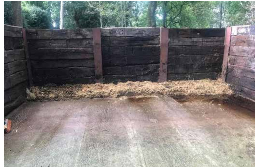
FIGURE 7: MUCK HEAP CONSTRUCT WITH NON-PERMEABLE BASE AND SIDES
