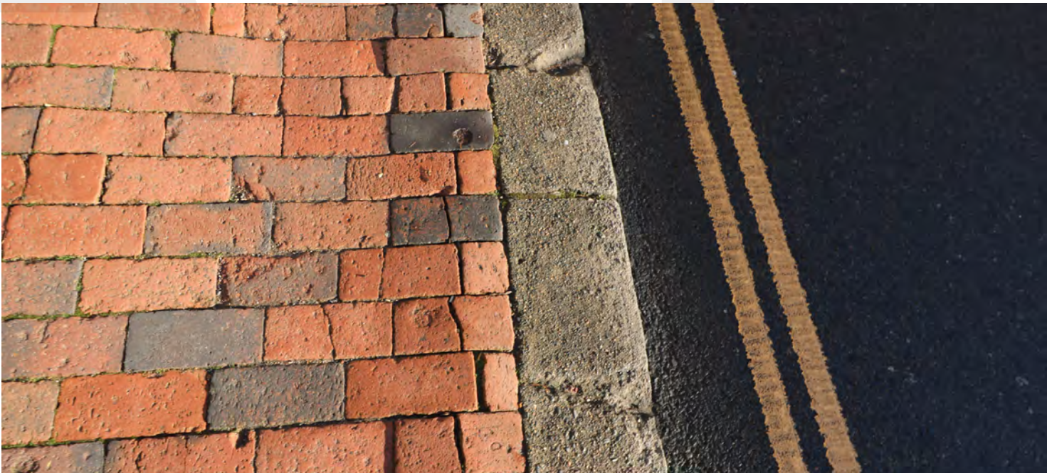
Figure 125: Characterful brick paving to the High Street with poor quality concrete kerbs
