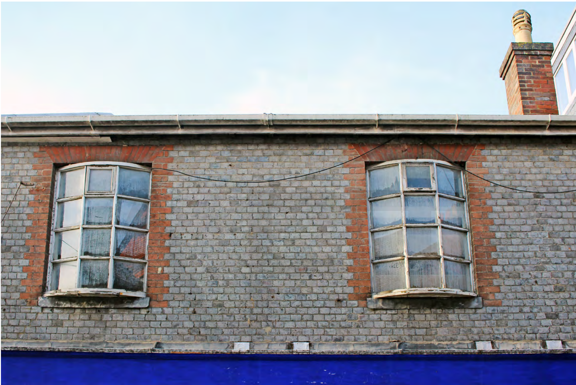
Figure 118: Non-original timber windows in disrepair
