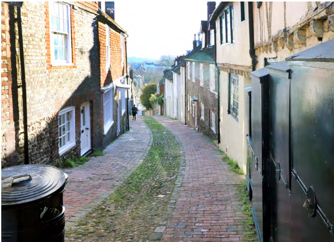
Figure 66: Cobbles and clay brick pavers to Keere Street
