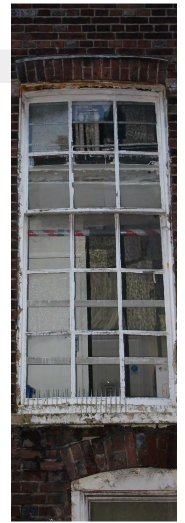
Figure 158: Pigeon spikes to the cill of a timber window in poor repair
