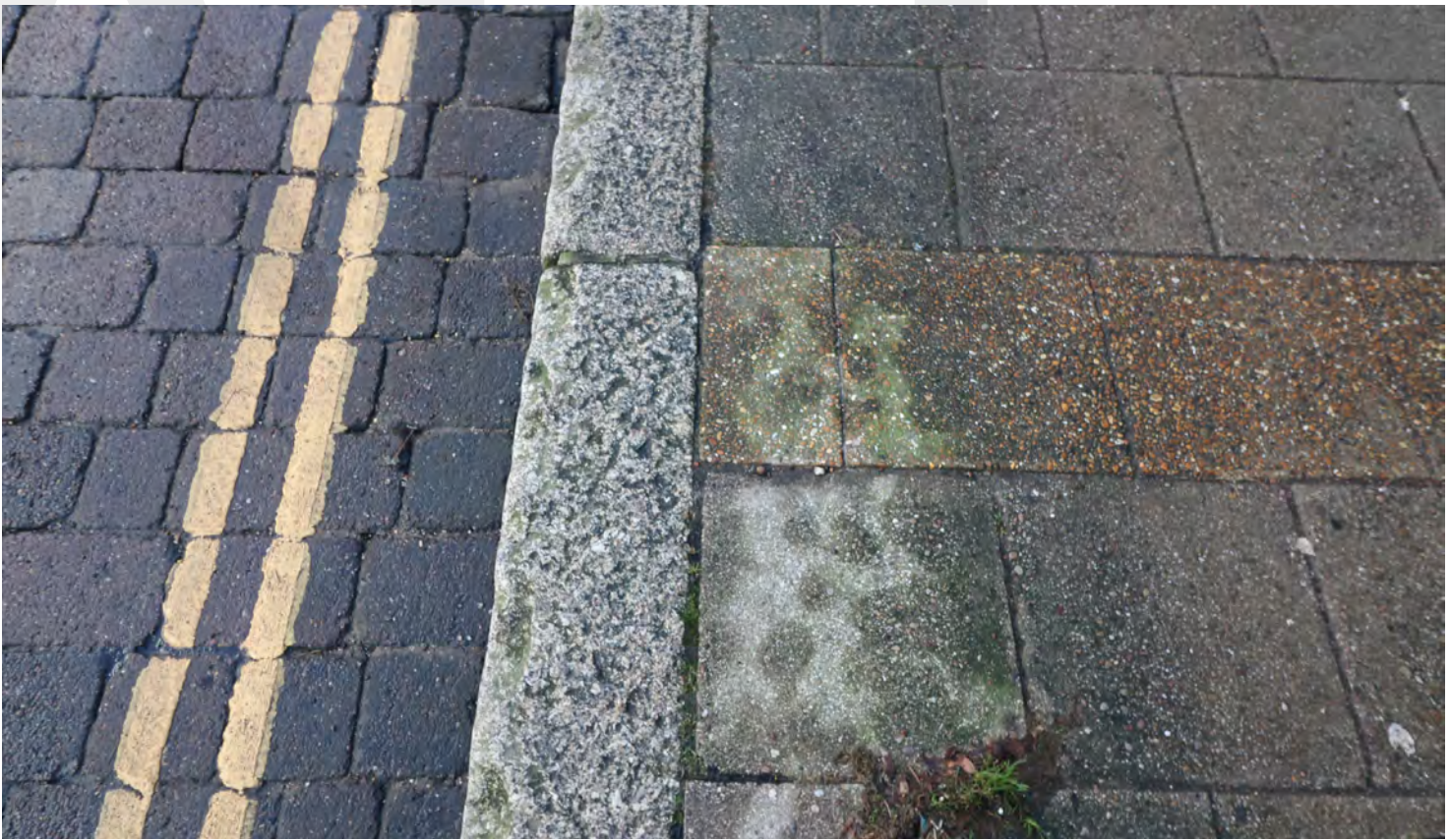
Figure 107: Modern concrete pavers to the High Street with traditional granite kerbs
