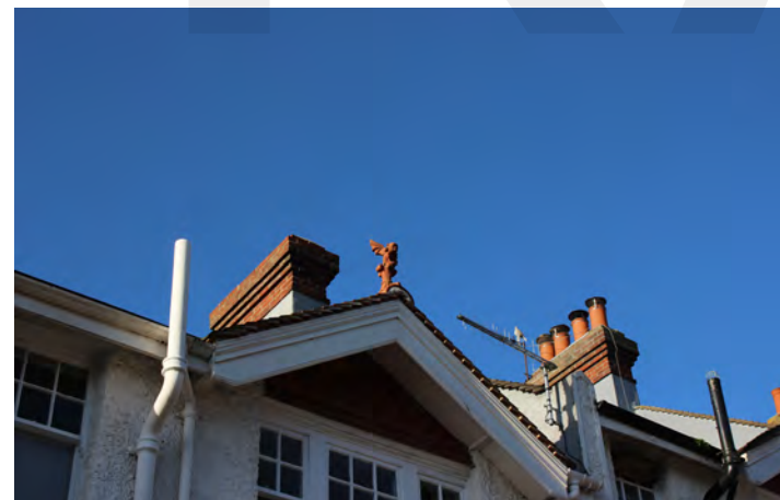
Figure 155: Cluttered drainage goods and TV antennae
