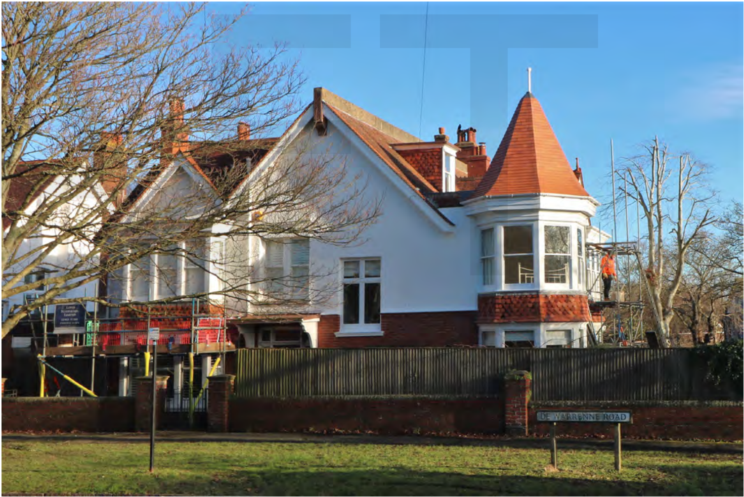
Figure 160: House in the Wallands during repair works, including the sympathetic reroofing of the corner turret
