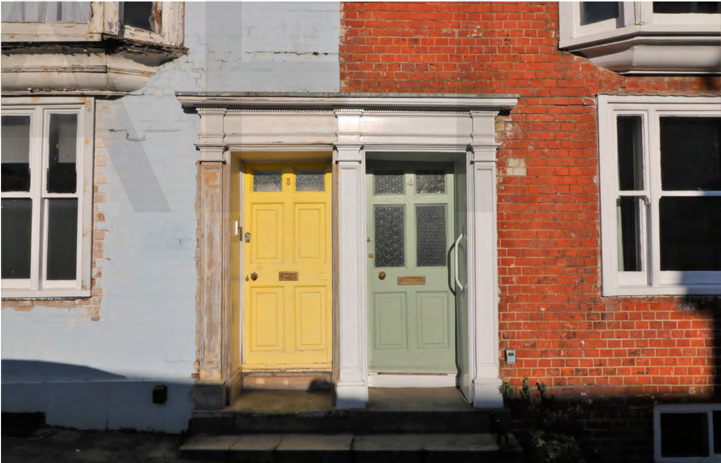
Figure 159: Neighbouring poorly-maintained and well-maintained houses, showing the impact of a lack of regular painting and maintenance on timberwork
