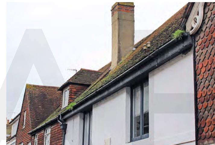
Figure 154: Vegetation growing in a blocked gutter on Cliffe High Street
