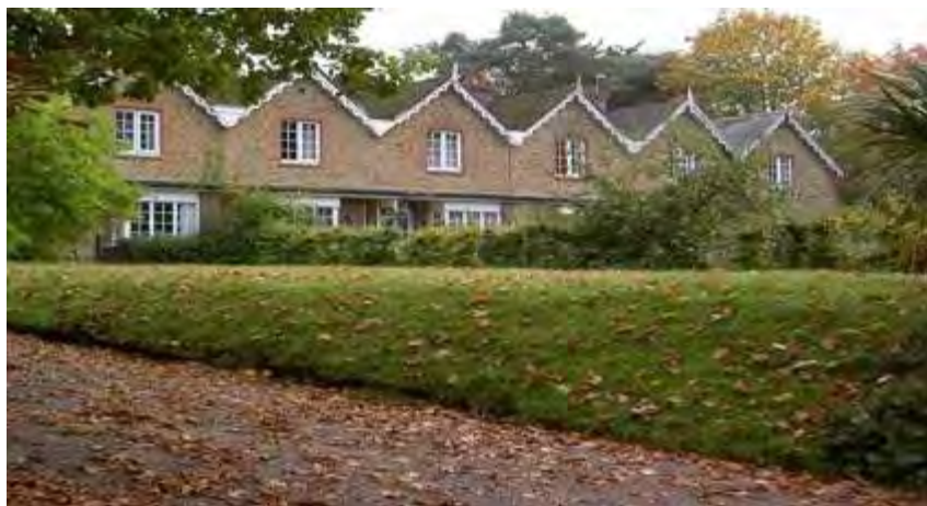
Rockpit Cottages, Rake Road
