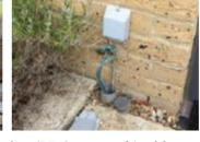
Figure 8.19: (left) Laying ducting (BT Openreach) with inspection chamber and (right) duct end with drawstring to allow for future easy laying of fibre cable to a house.
