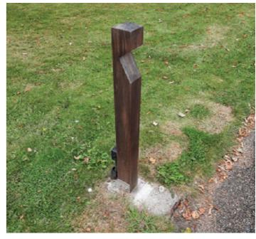
Figure 8.20: Simple timber bollard lighting directing light downwards in West Dean Estate.
