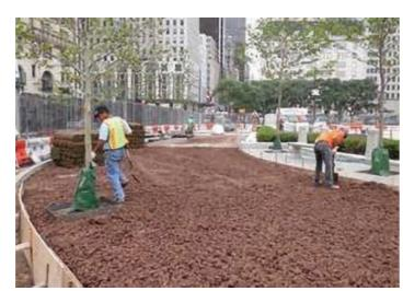
Figure 9.17: An example of a structural soil system (clean stone lattice with soil added) in New York City (CU-Structural Soil).
