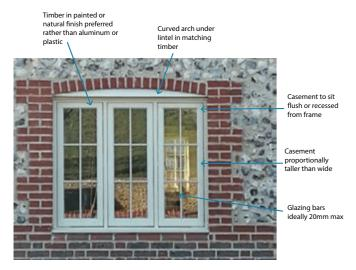
Figure 13.19: Acceptable detailing for traditionally inspired casement windows.
