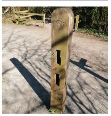
Figure 8.11: Timber cycle locking post on Centurian Way, West Dean.
