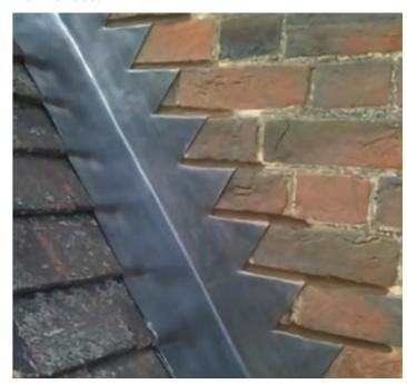
Figure 12.30: Good quality flashings in a roof junction.
