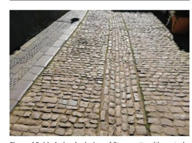
Figure 12.44: A simple design of Stone setts with central channel and blue, clay paver side detail make a beautiful place in a Petworth pedestrian street. The uneven texture may cause problems for some users.
