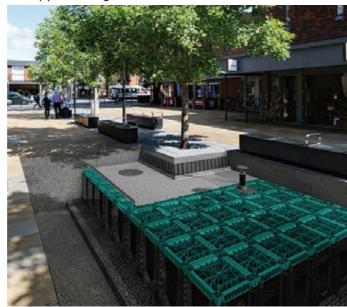
Figure 9.16: An example of a cellular system under a street (GreenBlue Urban).
