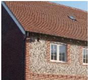
Figure 13.13: Exposed rafter feet with eaves ventilation between them on medieval building in Southampton and in a new development in East Dean.
