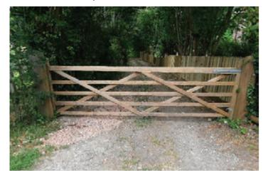
Figure 12.31: Five bar timber field gate, Easton.
