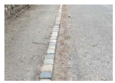
Figure 12.50: Setts are used to define the footway in Selborne.
