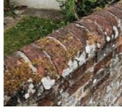
Figure 12.7: Two examples of traditional brick cappings in Tywford.
