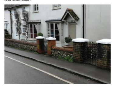
Figure 11.4: Front garden walls in Buriton in local stone (flint) and brick with pedestrian gates.
