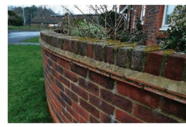
Figure 12.8: Traditional tile creasing in brick wall coping detail, in modern Midhurst development.
