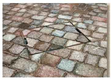
Figure 8.17: Service manhole recessed cover helps to protect integrity of paving, even when at an angle. (Pavingexpert.com).
