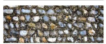
Figure 12.12: Galleted flint (flint shards incorporated into the mortar).
