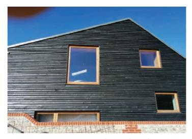
Figure 12.27: A contemporary designed new home in rural West Sussex uses dark stained horizontal timber cladding which references a locally common agricultural building material.
