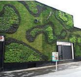
Figure 9.35 and 9.36: supported ivy green wall and intensive green wall.
