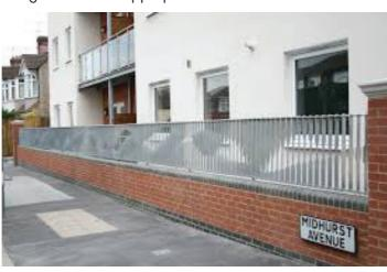
Figure 12.36: Newly built brick and simple galvanised railing boundary structure in a contemporary style development.
