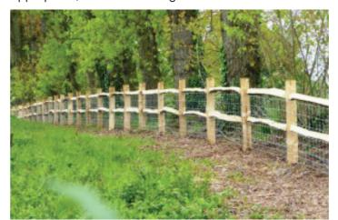
Figure 12.38: Chestnut cleft post and rail fencing with wire mesh animal proof fencing attached.
