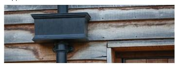
Figure 12.29: Aluminium rainwater goods (Guttercrest).
