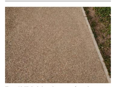
Figure 12.57: Resin bound aggregate footpath.
