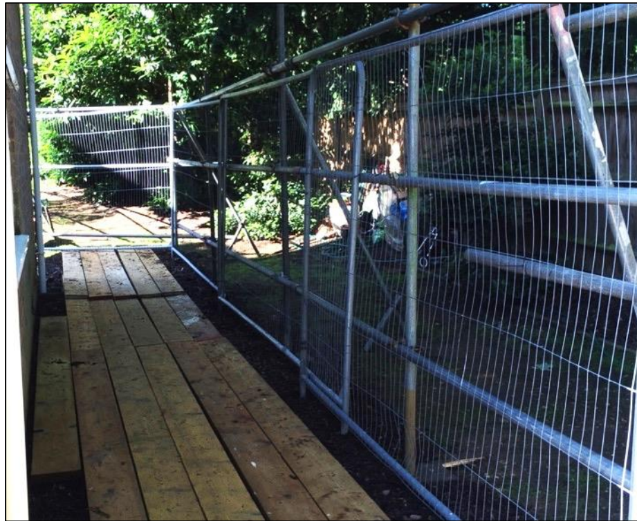
Scaffold board pedestrian ground protection
