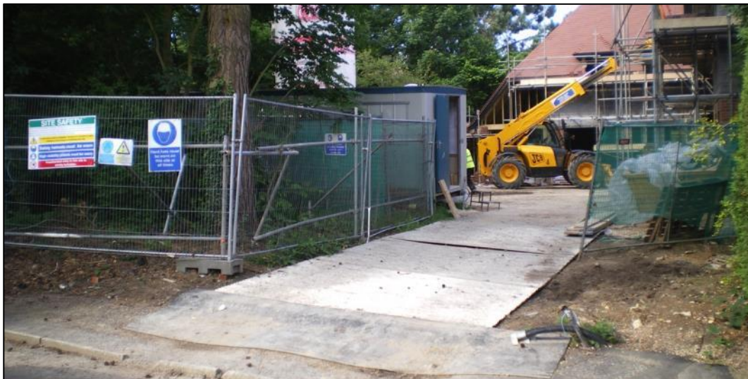
Vehicular ground protection trackway
