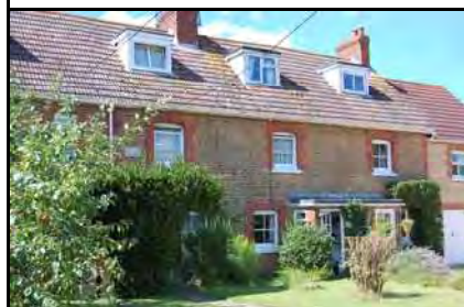
Carstone from the Lower Greensand used in a terrace in West Liss. Westernmost distribution of this material's use in Hampshire.
