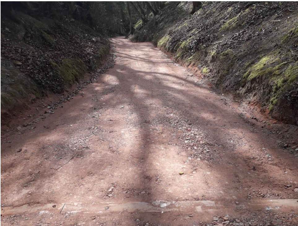
Photo 2: Byway Hawkley 745 following restoration work. Photo curtesy of HCC.
