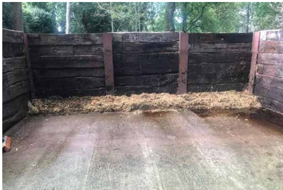
FIGURE 7: MUCK HEAP CONSTRUCT WITH NON-PERMEABLE BASE AND SIDES
