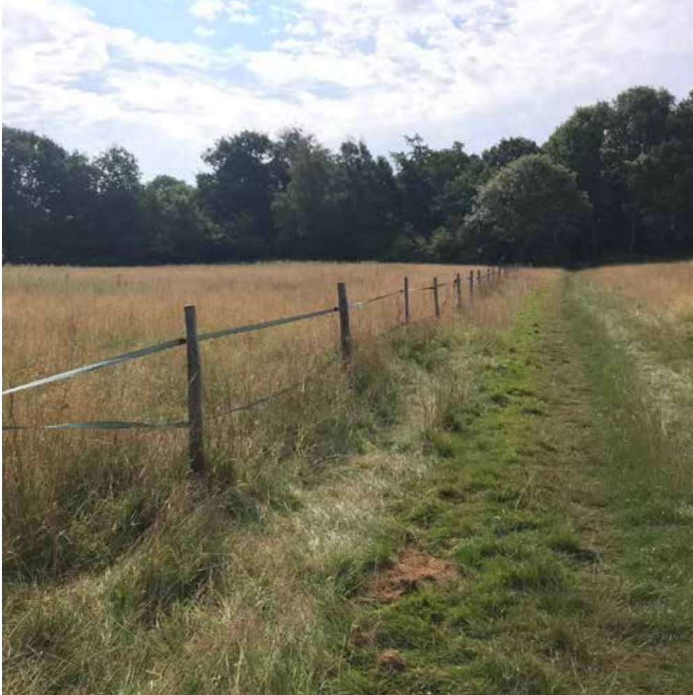
FIGURE 5: VISUALLY PERMEABLE FENCING USING TAPE
