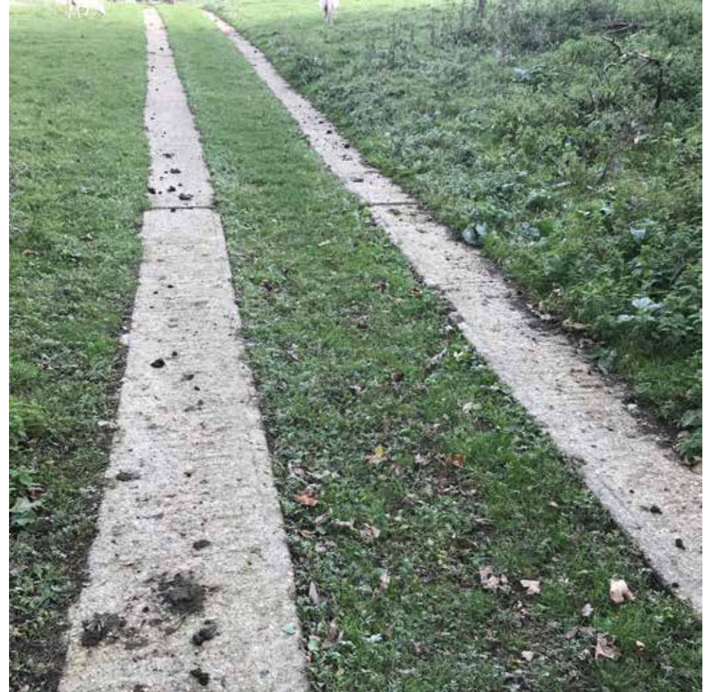
FIGURE 6: NARROW AND INFORMAL TRACK
