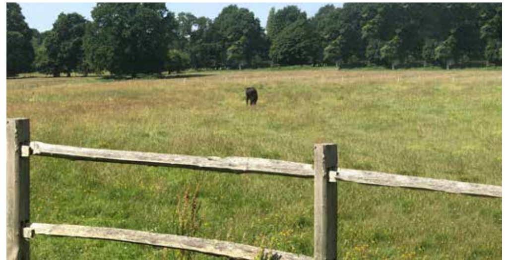
FIGURE 3F: HAND-CLEFT CHESTNUT FENCING (LOW WEALD)
