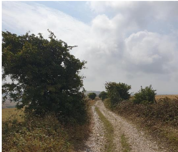
Figure 5: Track at Truleigh hill made of limestone and chalk with soft verges and no edges.
