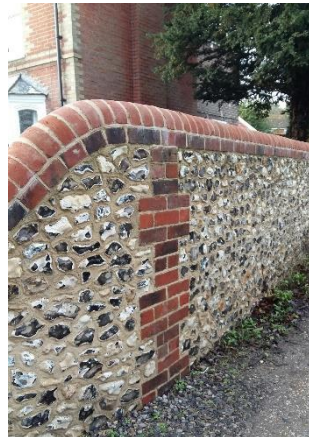
Figure 8 Brick and flint wall in the SDNP
