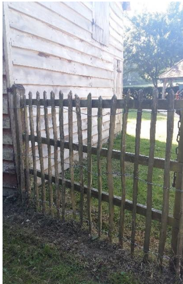
Figure 9 Chestnut pale fence in the SDNP
