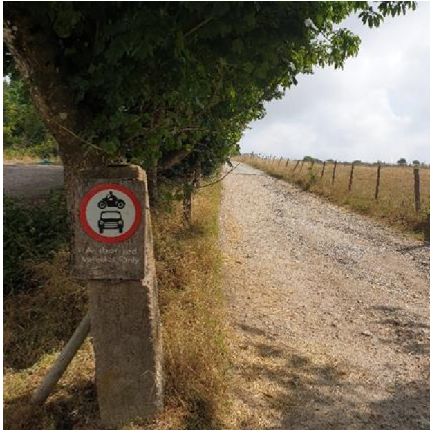
Figure 16 Road sign mounted on a wooden board and fixed to an existing fence post
