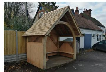
Figure 8.26: An attractive bus shelter in Selborne with a traditional timber construction and timber shingle roof.
