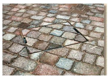
Figure 8.17: Service manhole recessed cover helps to protect integrity of paving, even when at an angle. (Pavingexpert.com).
