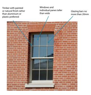
Figure 13.20: Acceptable detailing for traditionally inspired sash windows.
