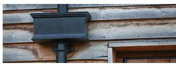
Figure 12.29: Aluminium rainwater goods (Guttercrest).
