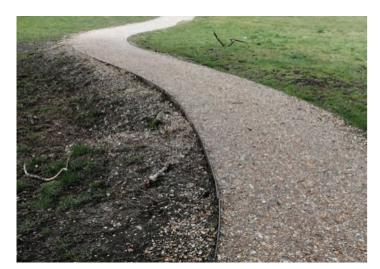
Figure 12.52: Steel edge details can also describe elegant curves in a subtle way and are more robust and long lasting than timber. Compacted stone footpath in Hampshire park.
