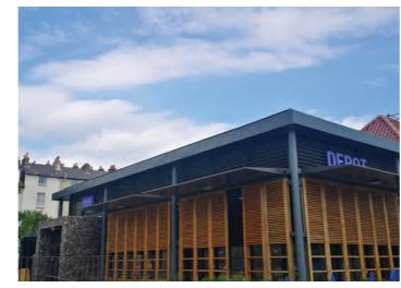
Figure 15.2: The Depot in Lewes uses external blinds to mitigate the effects of large windows at night.
