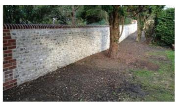
Figure 12.9: A well built, new flint wall with masonry piers and coping.
