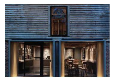
Figure 12.25: Horizontal timber cladding used in a contemporary building (Ditchling Museum of Art and
