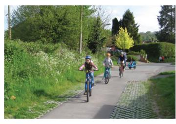
Figure 12.40: Reinforced grass paving used in Buriton to visually narrow the road while allowing for occasional wide vehicles.
