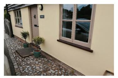
Figure 12.23: House in Hambledon showing how render is protected from ground splash back with brick detail.
