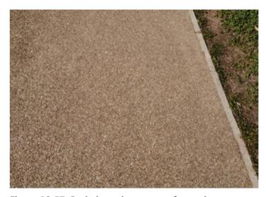
Figure 12.57: Resin bound aggregate footpath.
