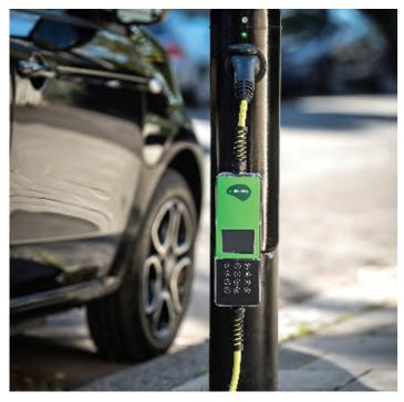
Figure 8.28: A converted lamp post housing an on street EV charge point (Lucy Zodion).
