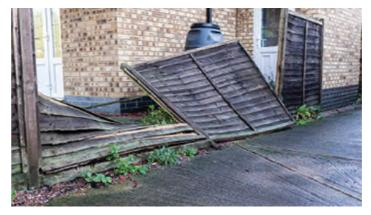
Figure 11.2: Poor quality and lightweight timber panel fences are not a good long-term solution in the public realm as they are not very robust.
