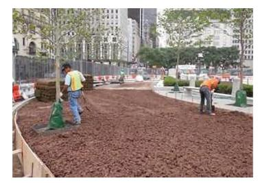
Figure 9.17: An example of a structural soil system (clean stone lattice with soil added) in New York City (CU-Structural Soil).
