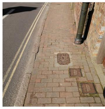
Figure 12.46: Concrete block pavers (here 'Tegula' in Petworth) are widely used in more urban contexts. This can lead to an 'anywhere' character whereas local stone or clay pavers are preferable as they reinforce local character.
