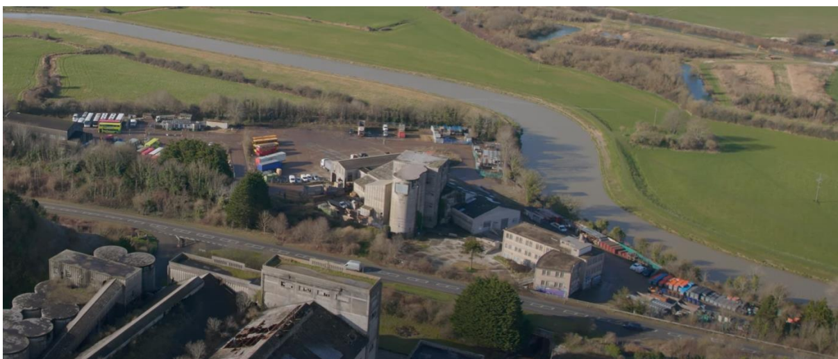
Figure 4.1: The Riverside looking west
