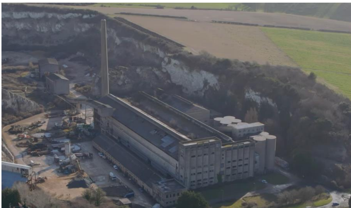
Figure 4.2: The Cement Works looking south east
