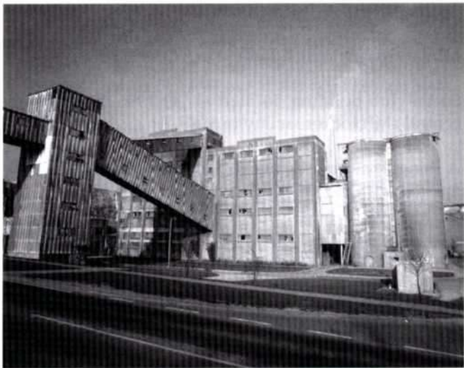
Fig. 15 West elevation of kiln house and coal store with overhead conveyors (demolished in 1995) [Jacob Purchase]
