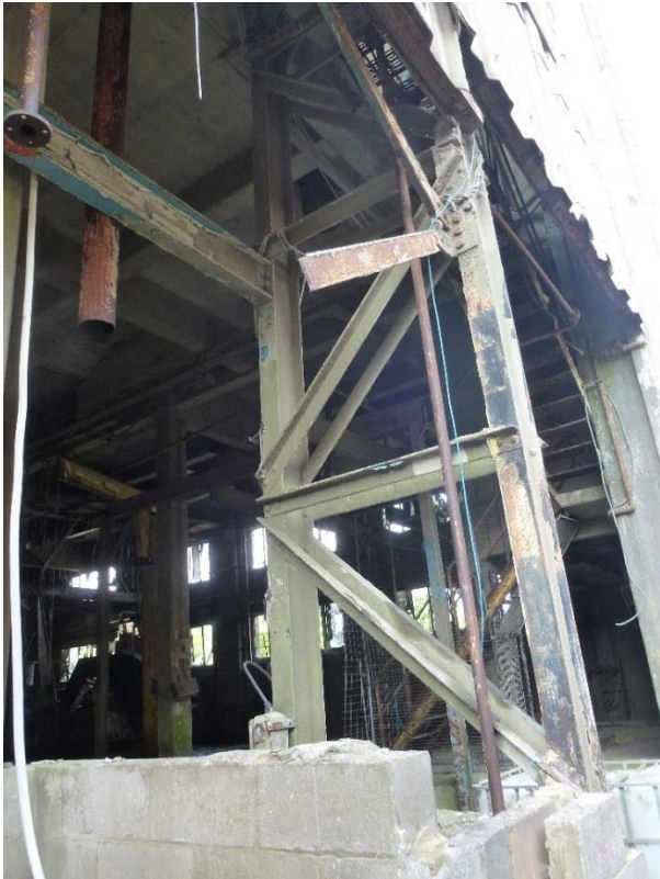
Photograph 13 - Severed Kiln House bracing.
