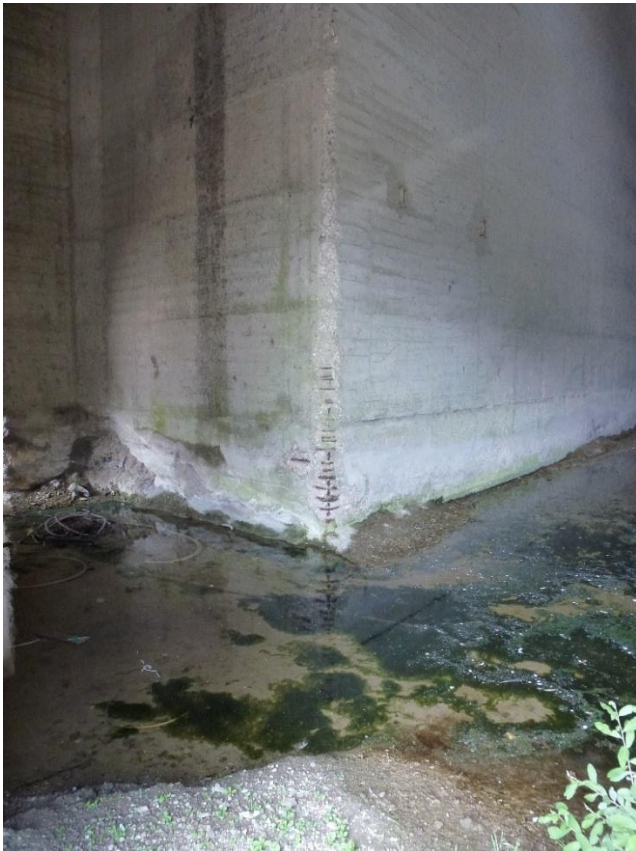
Photograph 19 - - Concrete spalled from Clinker Store wall.
