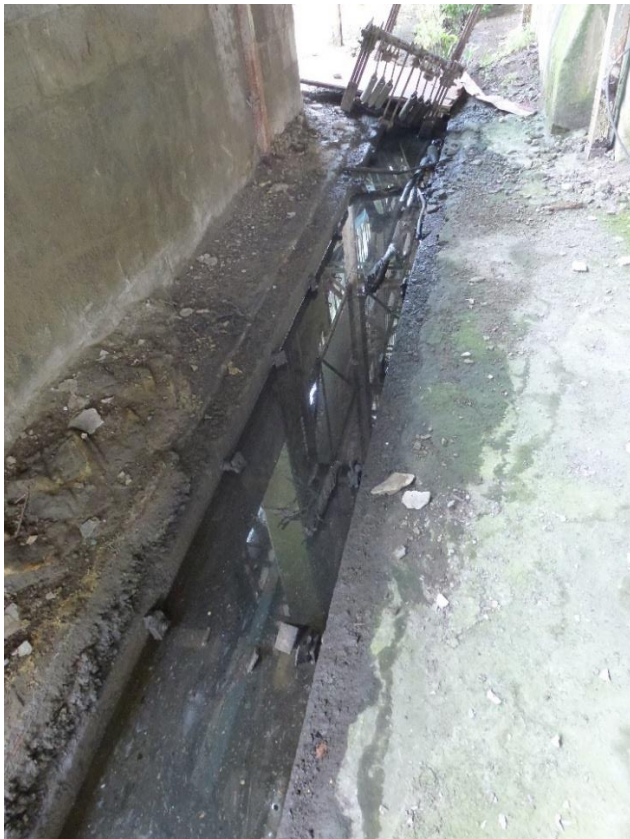
Photograph 14 - Damaged Kiln House floor ducts.
