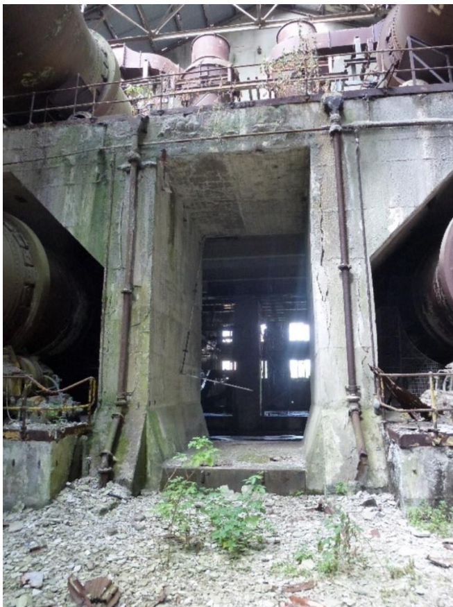
Photograph 7 - Cracking to concrete piers in the Kiln House.
