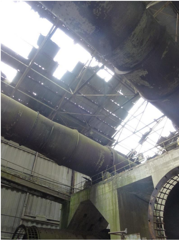
Photograph 15 - Damaged Kiln House roofing - rotary kilns and piers in foreground.
