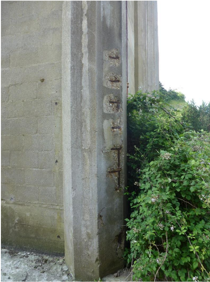
Photograph 5 - Concrete framed structure at front of Kiln House - spalling to spandrels.
