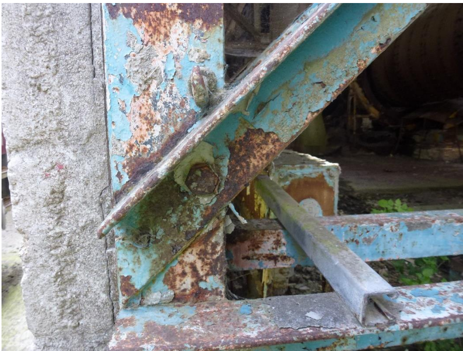
Photograph 11 - Superficial corrosion of Kiln House steelwork.
