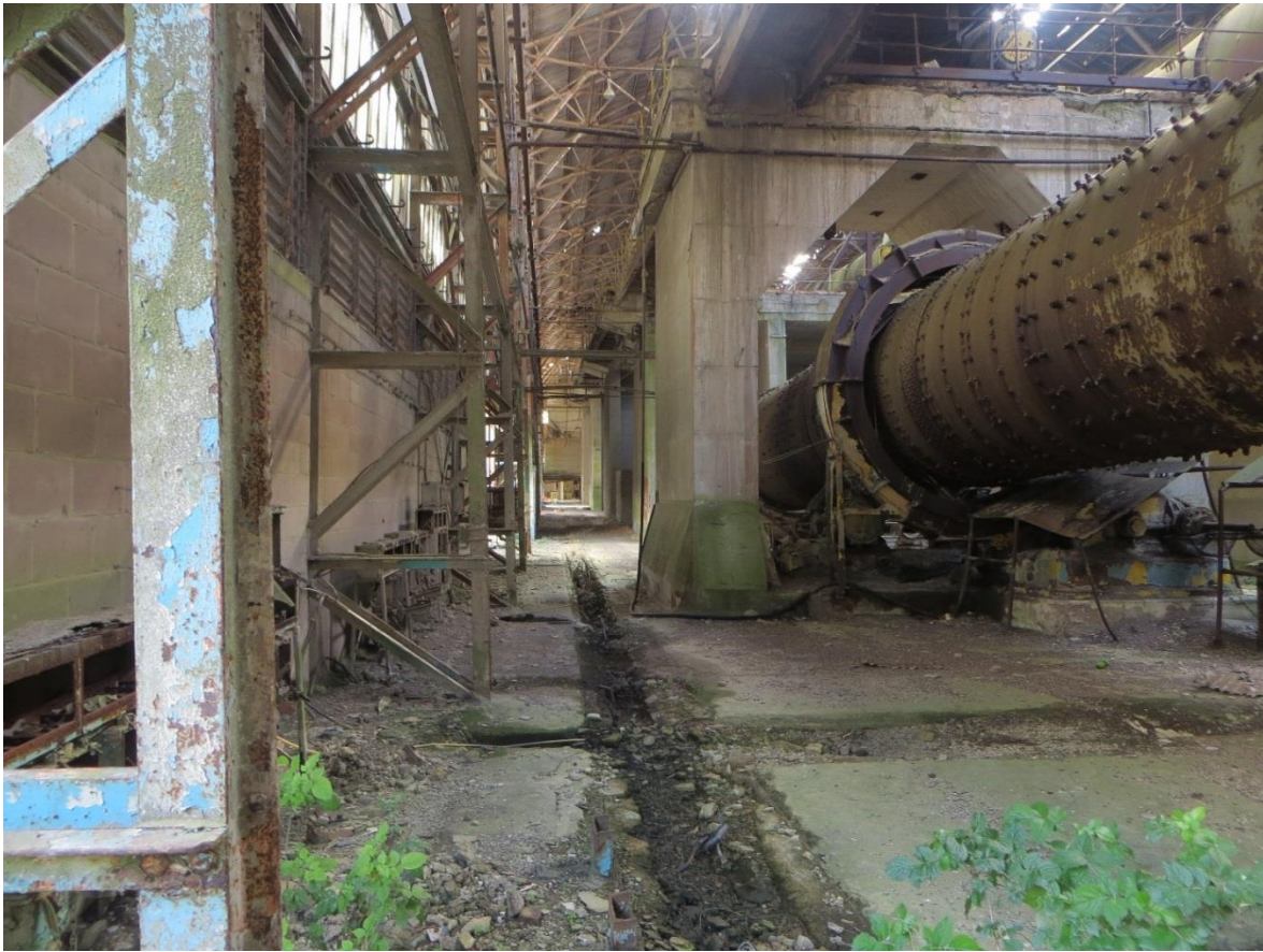
Photograph 21 - Kiln House, corroded steelwork, damaged floor slab.
