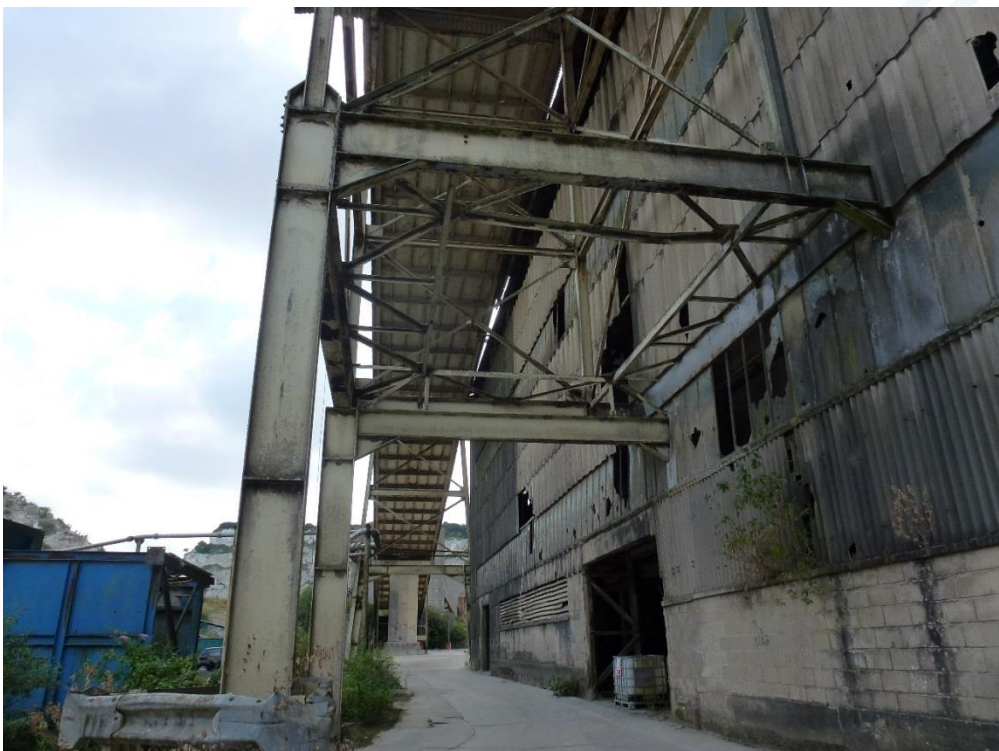
Photograph 16 - Failed Kiln House cladding - eroded blockwork, superficial external steelwork corrosion.
