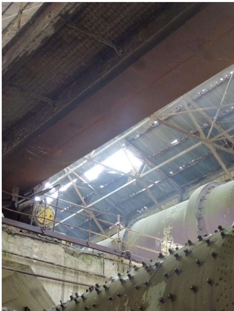
Photograph 12 - Failed Kiln House roofing.
