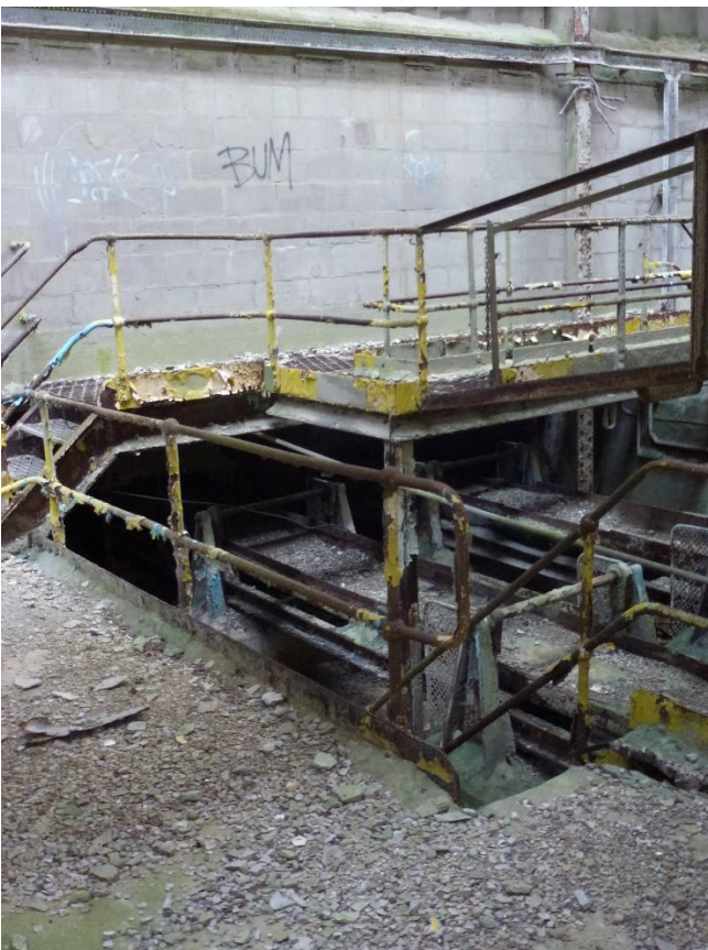
Photograph 20 - - Corroded ancillary steelwork.
