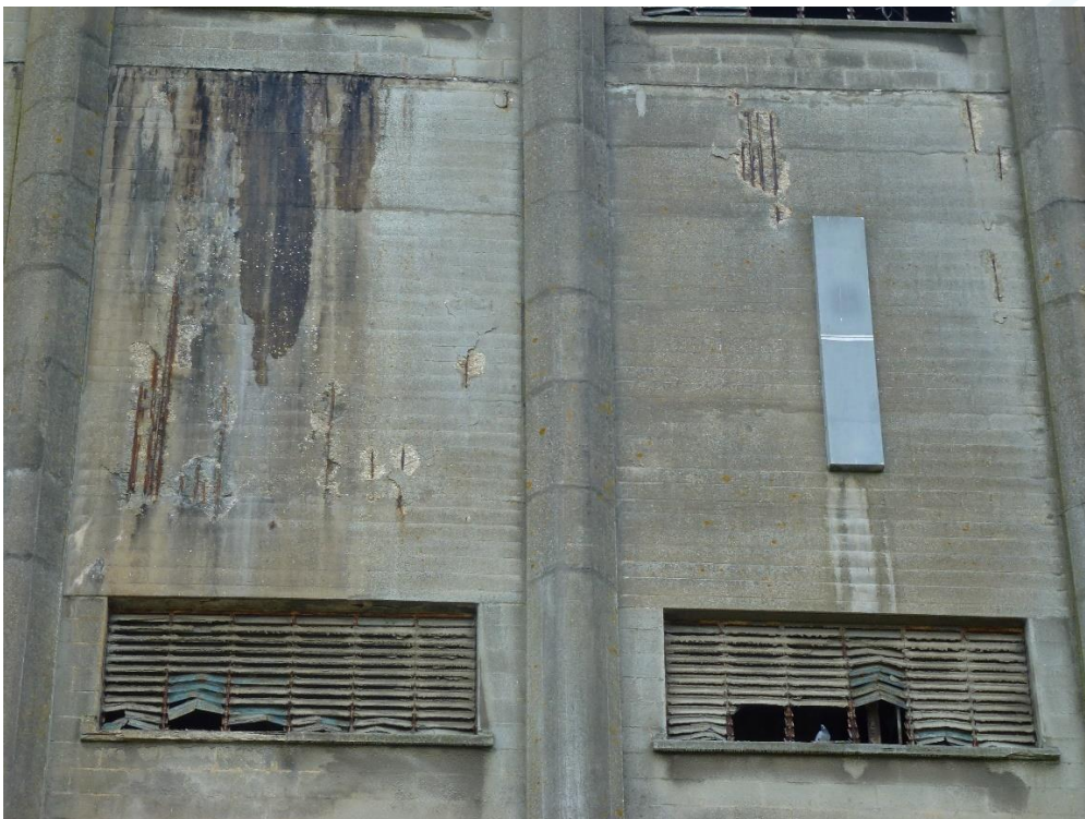
Photograph 5 - Concrete framed structure at front of Kiln House - spalling to spandrels.
