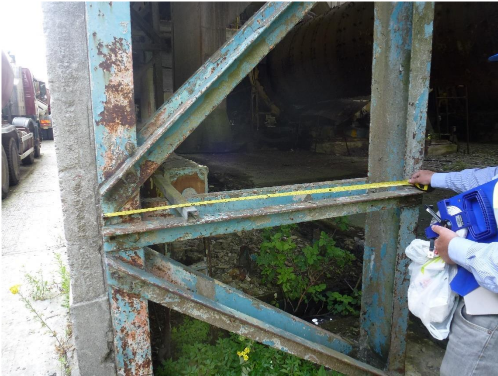
Photograph 6 - Superficial corrosion of Kiln House stanchions.
