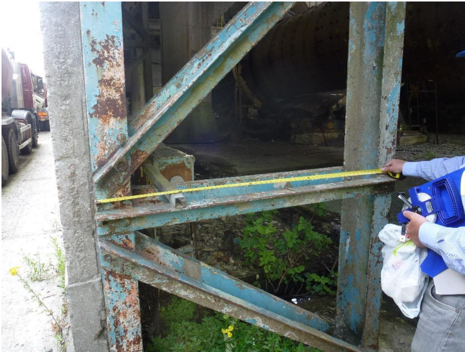
Photograph 10 - Superficial corrosion of Kiln House steelwork.
