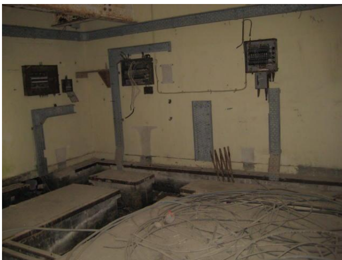
Plate 51: Kiln Shed – electrical equipment has been stripped and removed
