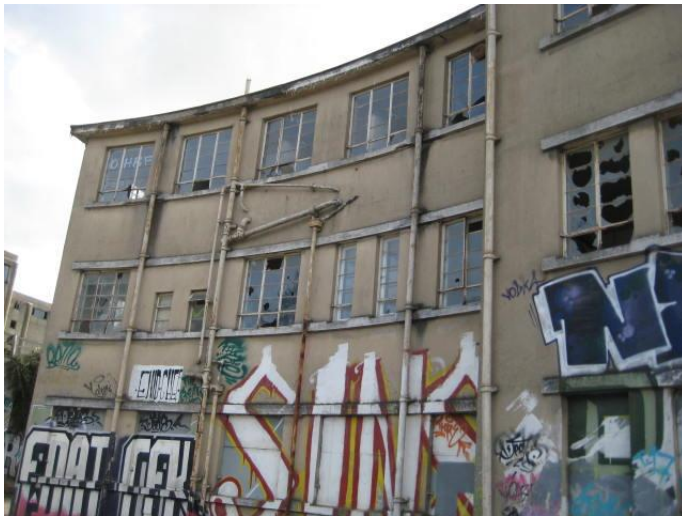
Plate 2: Former Admin and Laboratories Block
