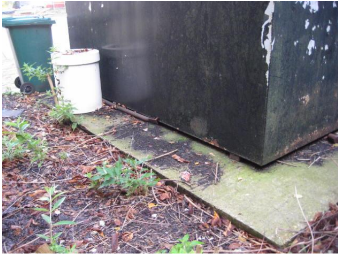
Plate 41: Handling Shed (adjacent to Generator House)
