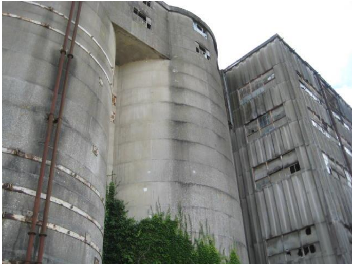
Plate 5: Service Road to Storage Buildings
