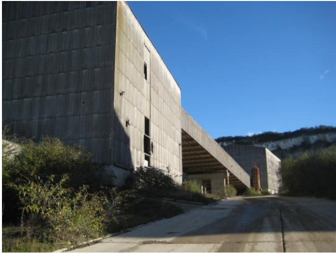
Plate 68: Tarmacadam processing in yard area
