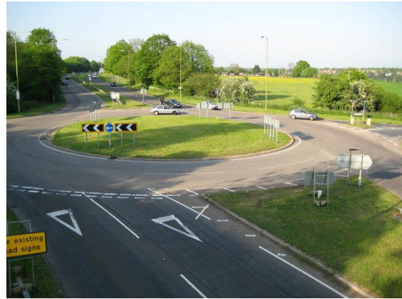
Four-arm roundabout to improve access entering and exiting the site on the A283. (Credit: Nigel Cox)
