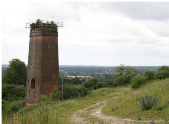
Betchworth Quarry: a former lime kiln, which has been retained to become a habitat for bats. (Credit: Hugh Craddock)
