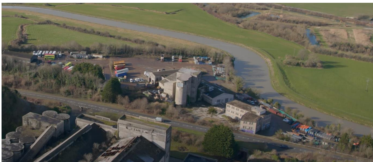
Figure 4.1: The Riverside looking west
