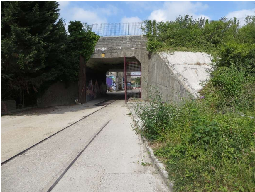
Figure 9-2: Vehicular underpass between Areas A and B
