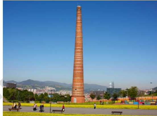
Parque Etxebarria, Bilbao: Retain the chimney and place it centrally in a green space on the site as a sculpture and to reference its industrial history. (Credit: Bilbao Turismo)
