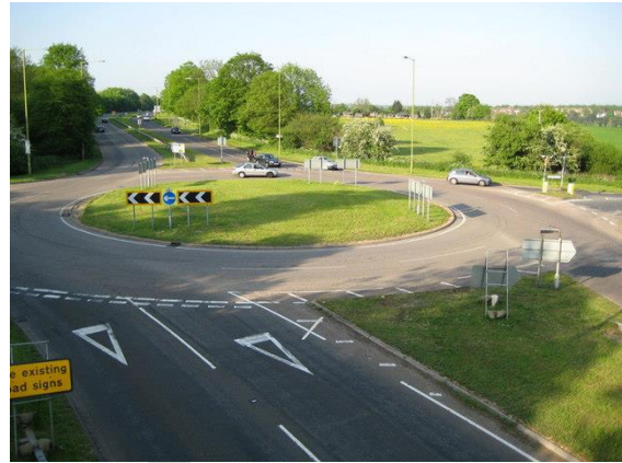
4-arm roundabout to improve access entering and exiting the site on the A283. (Credit: Nigel Cox)
