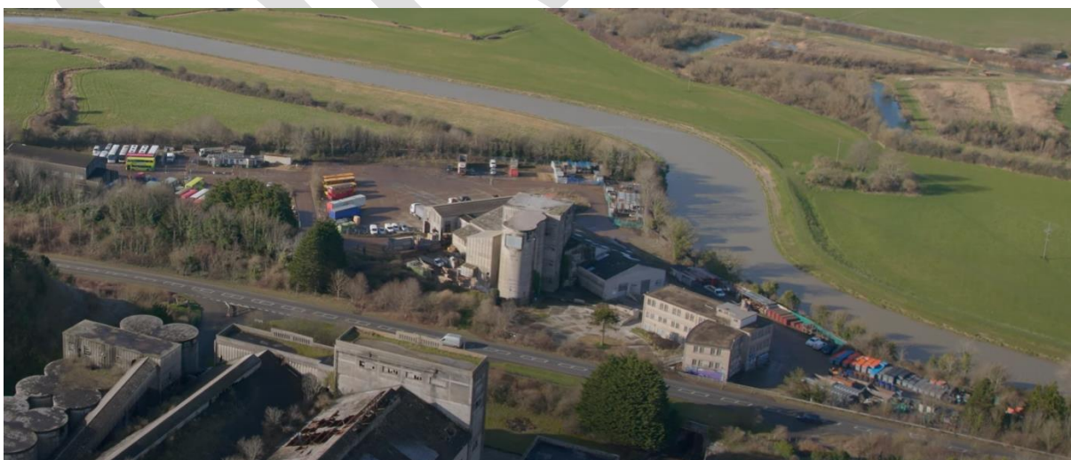
Figure 4.1: The Riverside looking west
