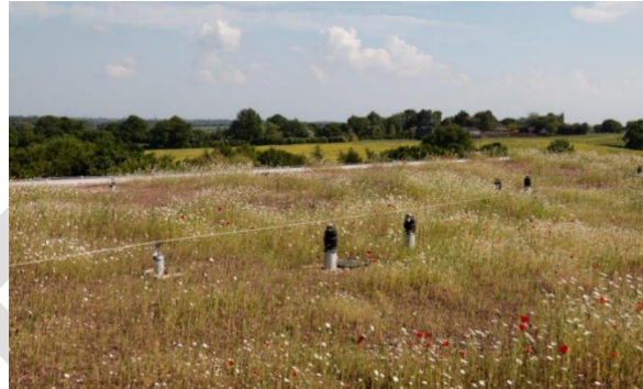
Biodiverse green roofs on residential and commercial buildings to mitigate runoff and provide habitat for various species (Credit: Susdrain)
