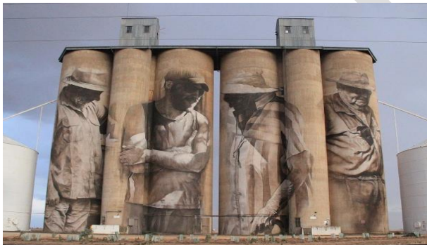
Buildings and infrastructure of cultural importance are retained and repurposed into a canvas for large scale artworks (Credit: Visit Victoria)
