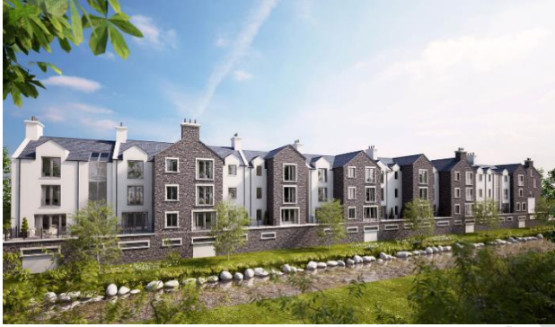
Riverside housing using colours that are in keeping with the landscape. (Credit: Oakland Holdings)
