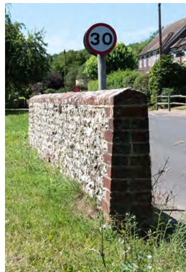
Left: Flint and brick wall Old Barn Crescent – good repair showing tapering profile of flint wall
