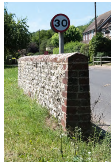
Left: Flint and brick wall Old Barn Crescent – good repair showing tapering profile of flint wall
