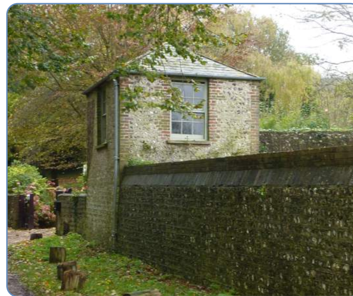
Figure 19: Grade II listed garden wall & gazebo at the Manor House
