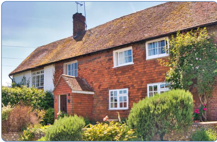
Figure 21: Hollowdown and Barn Close.
