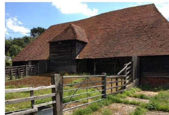
Fig 5: Grade II. listed threshing barn (north elevation) before conversion
