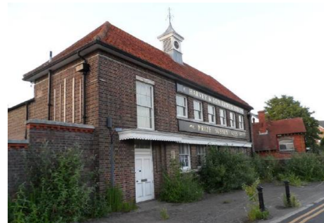
Fig 2: The original Depot building
