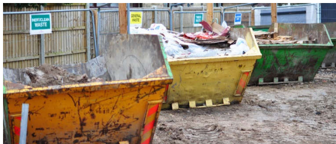
Segregated construction waste
