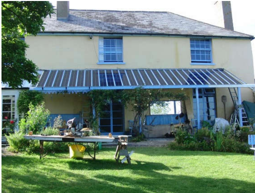
PV glazing in a discreet location
