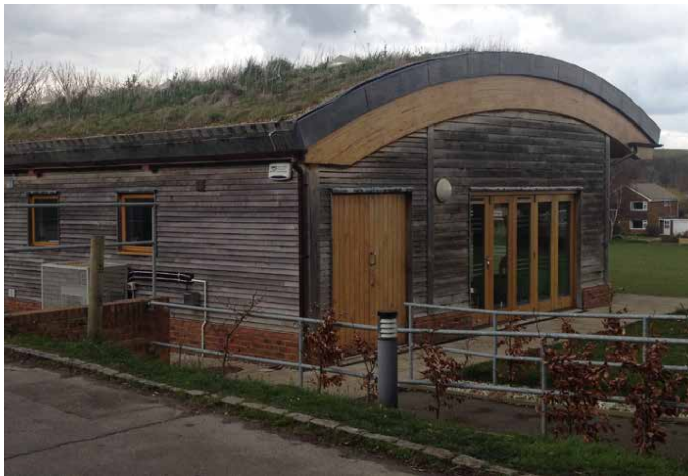
Photo of the green roof on Kingston Village Hall providing insulation for the building, rain water retention and habitat for wildlife. © V Craddock
