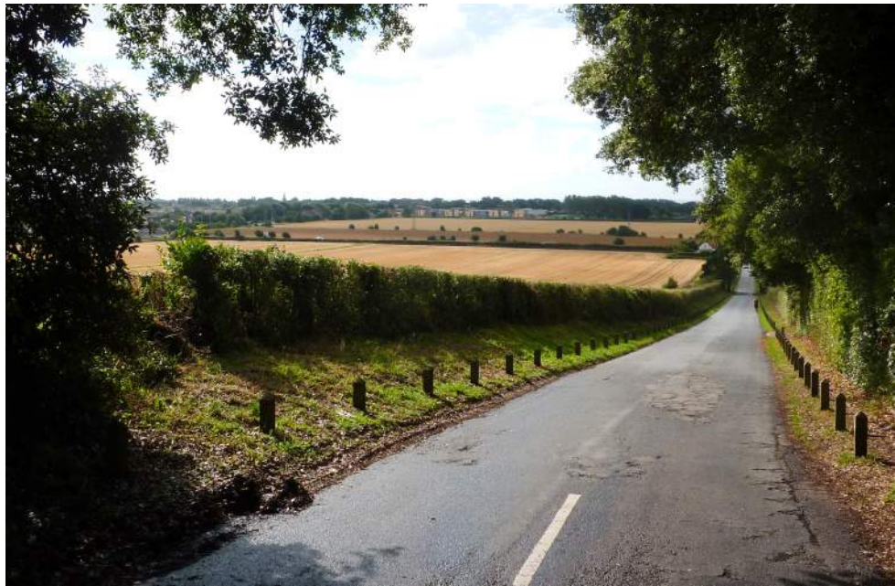
Figure 6: Views out from the Conservation Area to the surrounding landscape are few but the main exceptions is this view from the top of the drive. The poor condition of the road surface can be seen in the 'before' shot above and the improved surface in the 'after' photograph below.
