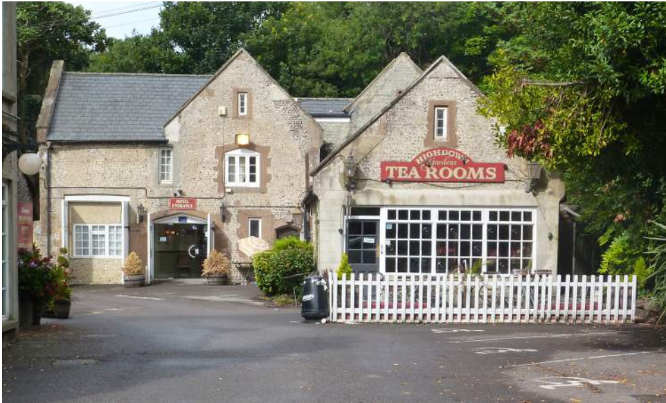
Figure 8: The Stables and Butler's and Carriage House, before the recent works (above) and after (below). In this case little has changed beyond the painting of the tea room window and the sign.
