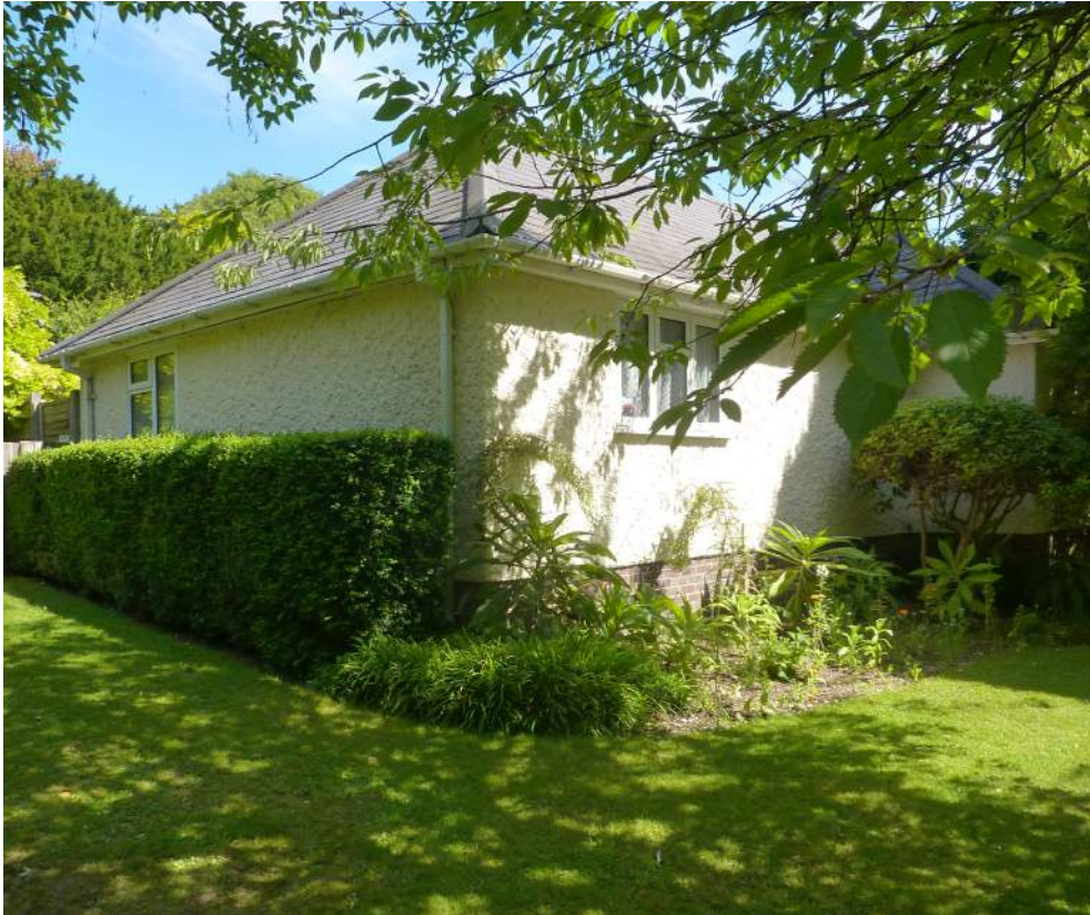
Figure 15: Bungalow within the garden built for James Buckman and formerly used as an office and mess room by the the gardening team. As part of the the Borough Council's project to enhance the garden, this will be extended and converted to form a new visitor centre.
