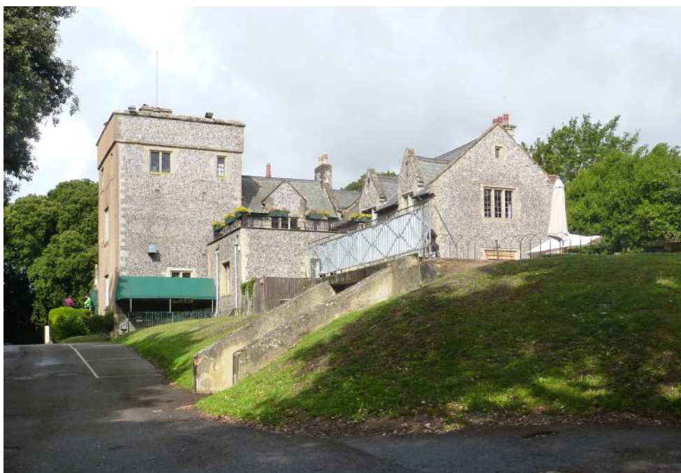
Figure 7: Highdown Tower from the south-east before (above) and below (after) the recent works. The removal of the green canopy and the painting of the railings have both improved the appearance and setting of the hotel
