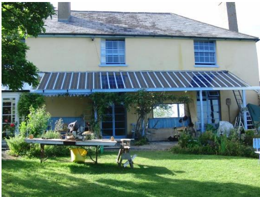
PV glazing in a discreet location
