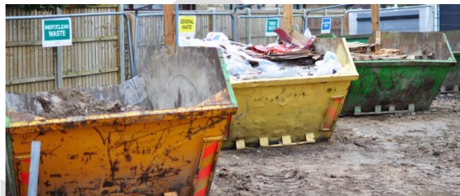
Segregated construction waste
