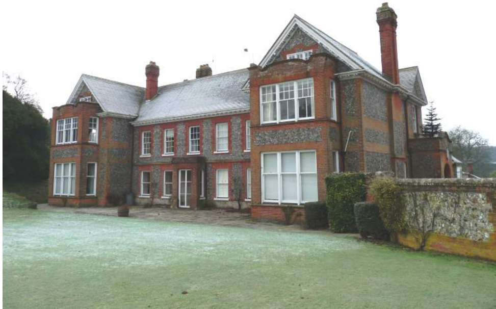
Figure 14 : Cissbury (above) is a Grade II listed building. The centre portion of the east front is an C18 farmhouse of two storeys and five windows in width. Gabled wings, each containing an attic window and with a large projecting bay of three windows on ground and first floors, were later added to the original building. The Lodge (below) to the main house sits at the entrance on Nepcote.
