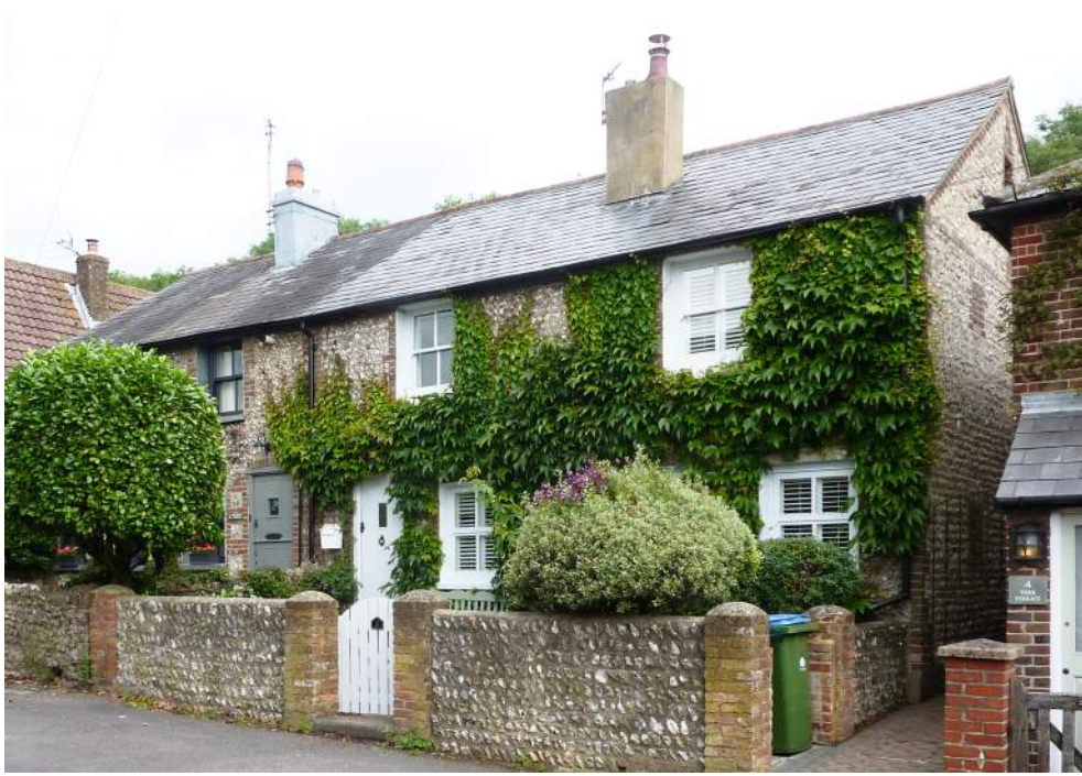
Figure 11: Further down Nepcote, Millbrook Cottages (above) and York Terrace (below) have also been modernised but have retained much of their historic character and continue to make a positive contribution to the character of the Conservation Area
