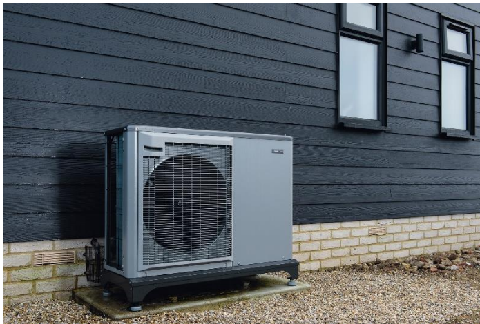
Air Source heat pump (Source: self-build.co.uk)
