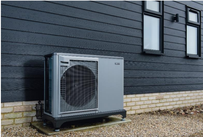
Air Source heat pump (Source: self-build.co.uk)
