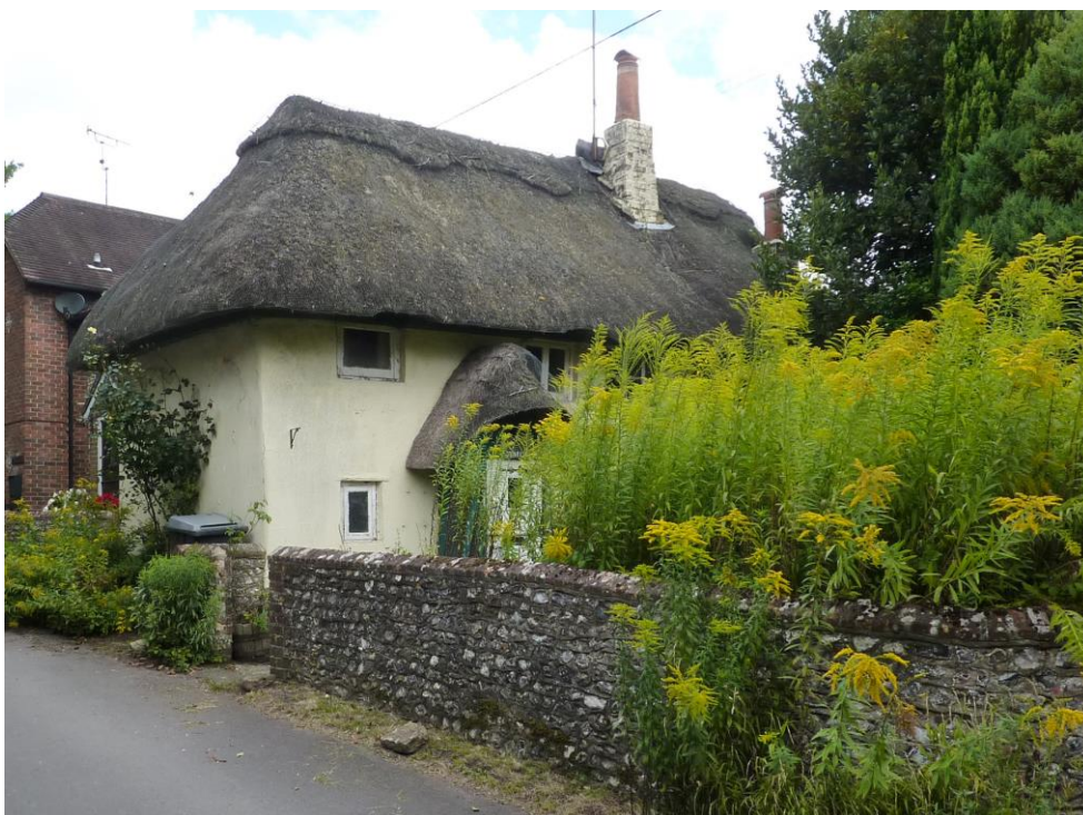
Figure 28: Sunrise ; an important survival of cob construction within the village and a building identified as 'vulnerable' in the National Park's Buildings at Risk Survey. The cottage has been recently re-thatched.
