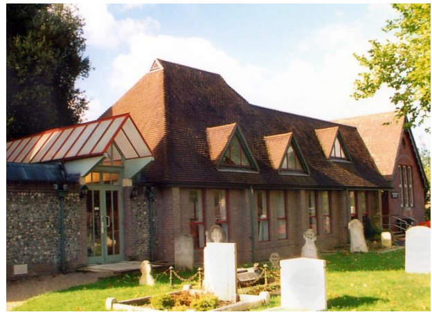
The Paterson Centre attached to the village church – sympathetically designed to match the original Victorian school schoolroom at the far end of the building
