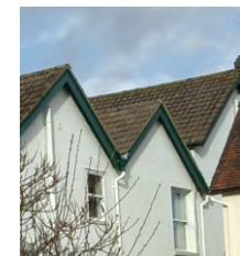
Centre valley gutters are found on many houses in Liss, either transverse or parallel to the front of the house. If they are to be emulated, then the valley must be carefully designed for regular maintenance and preventing the hopperheads from icing up when the snow in the valley starts the process of melt and freeze
