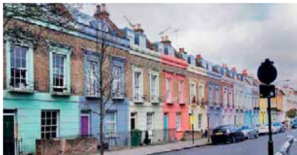
Coloured walls to improve the façade
