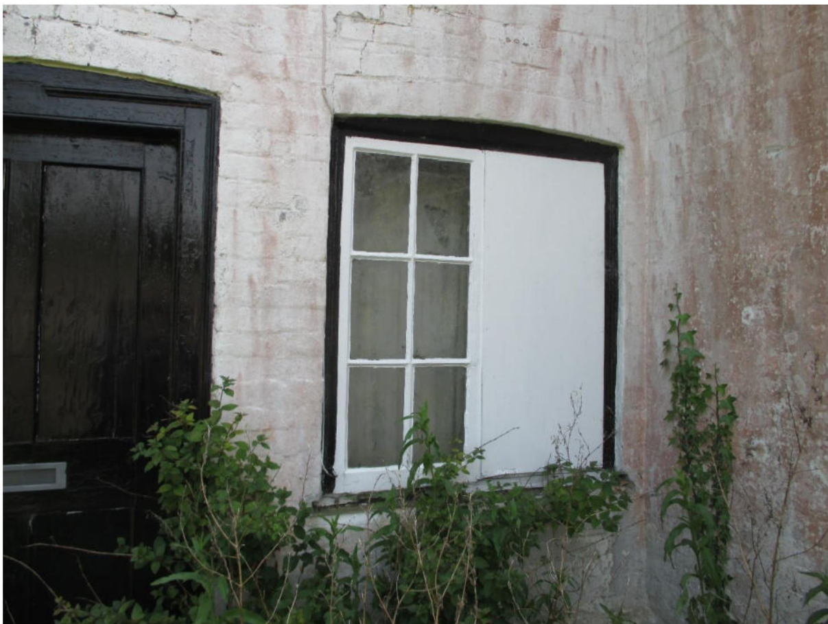
South Ground Floor Casement
