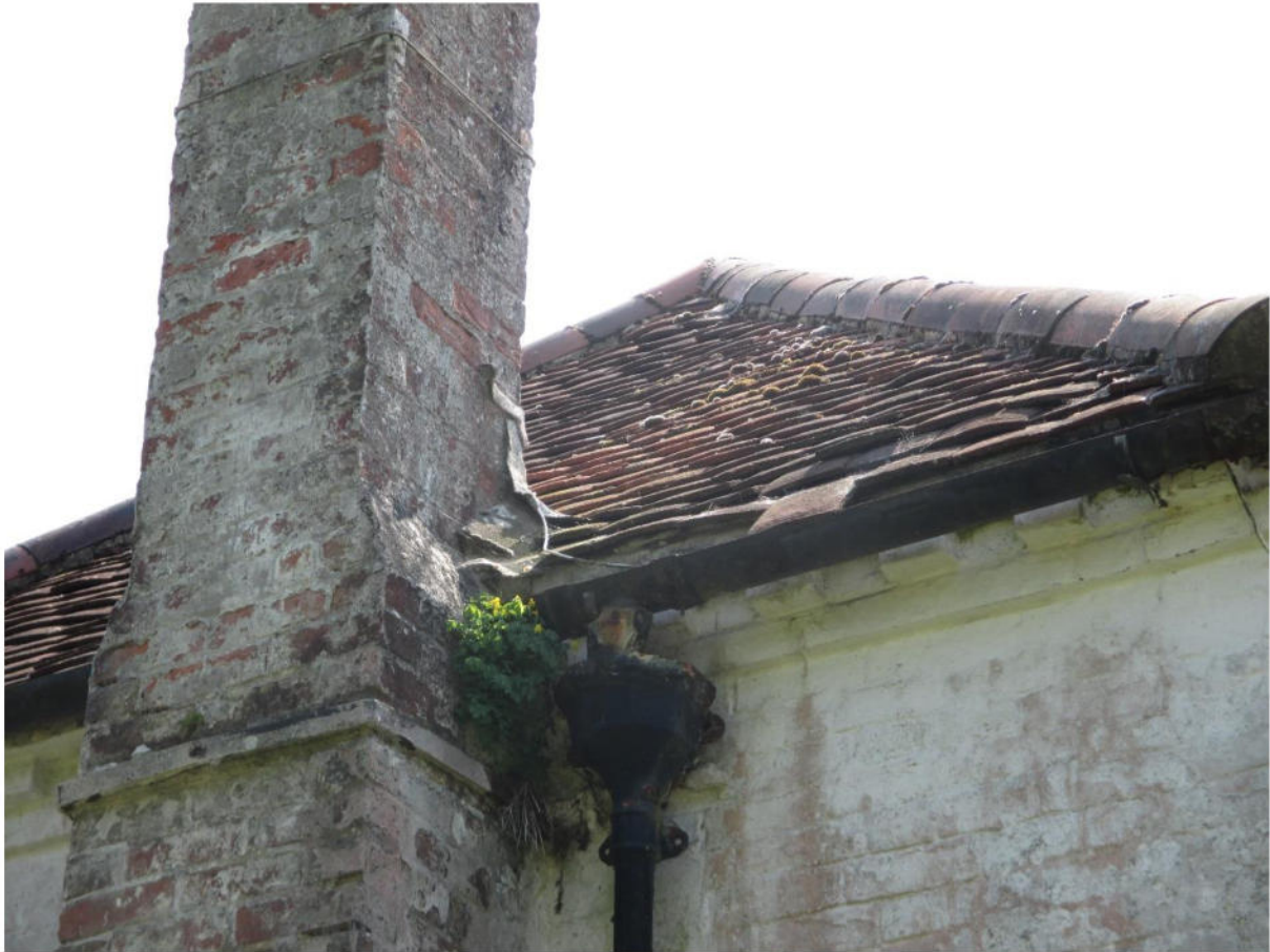
North Roof Pitch and Chimney Stack of Cottage
