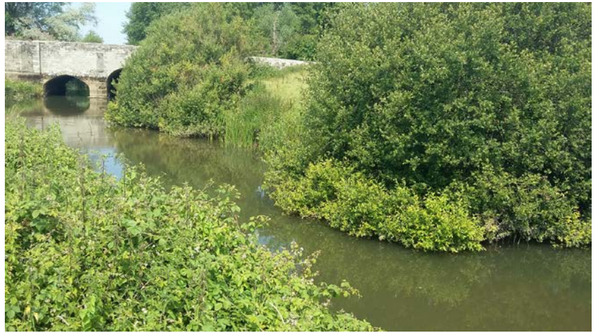
Fittleworth Bridge, River Rother
