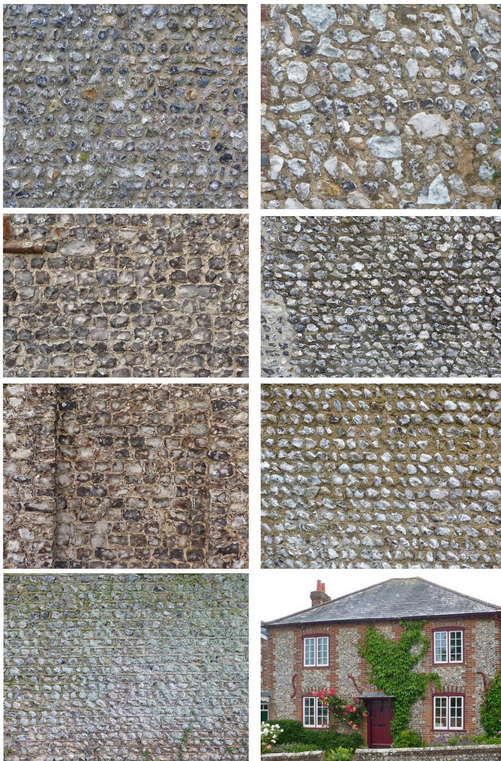
Figure 14: The appearance of the flintwork varies throughout the village; the panels above show some of this variety, which ranges from fairly rustic through to quite fine and includes some examples of galletting. The irregular nature of most flint requires the use of an alternative material to form corners. In Slindon this is almost invariably brick and it is often used in a distinctive fashion in which the brickwork jambs of the ground floor and first floor windows/ doors are continuous.
