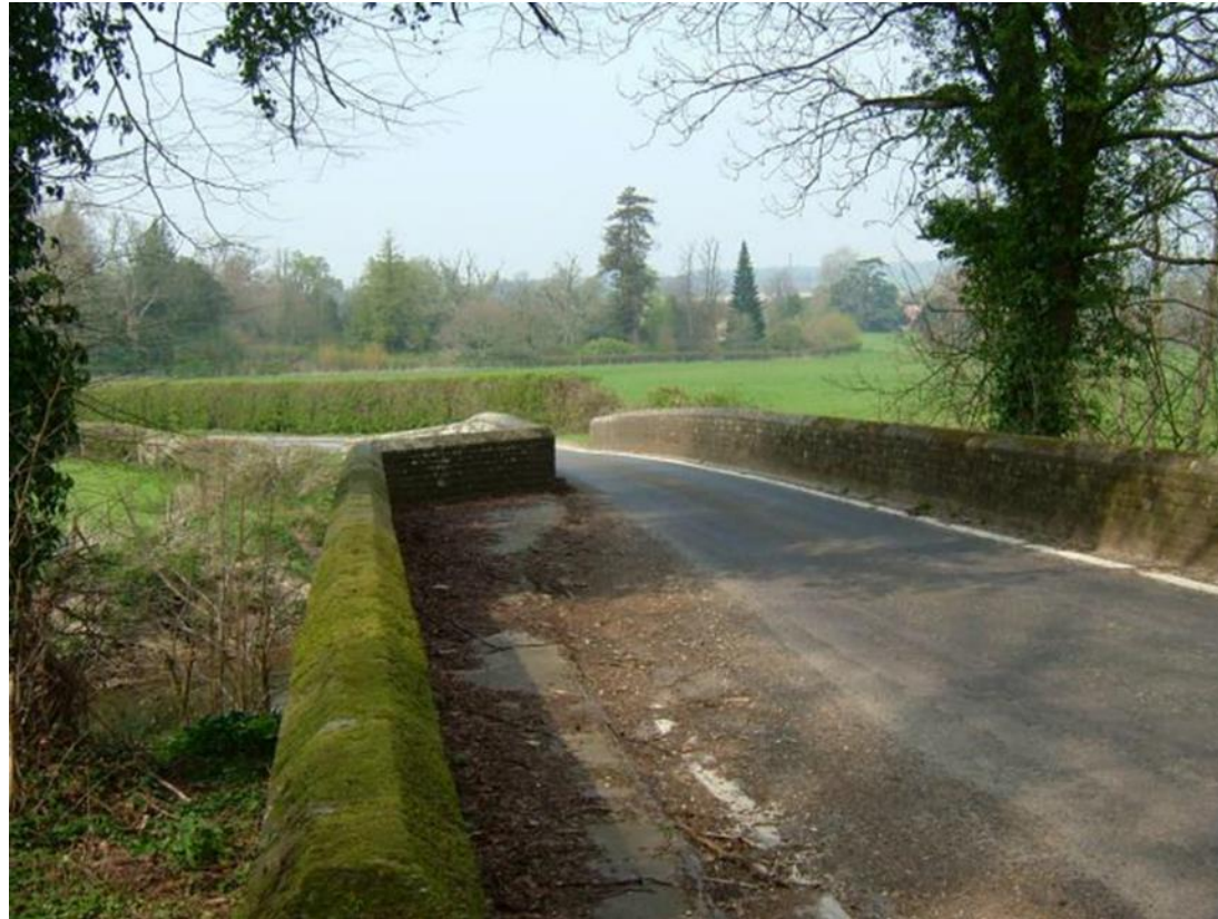
River Rother bridge, Woolbeding
