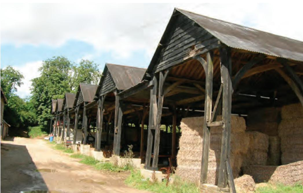
This shows a yard for covering ricks of hay and corn in north Berkshire, built in around 1900 of machine-sawn softwood with corrugated iron roofing. Photo © Sarah Orr
