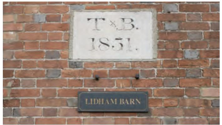
Flemish bond (alternate headers and stretchers in the same course) largely replaced English bond in the 18th century. These handmade bricks are more regular in size and the mortar joints thinner than earlier brickwork and the brickwork incorporates burnt headers, the dark bricks that were in the hottest part of the kiln. Burnt headers can be used as a decorative feature in the brickwork. Photo © Bob Edwards
