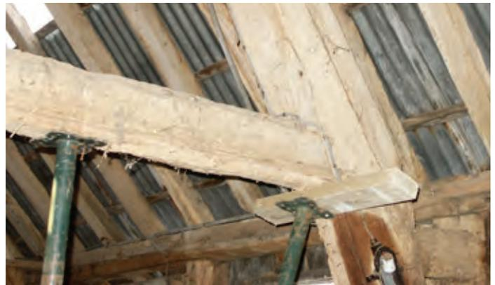
Evidence for vertical boarding. The butt-edged boards were set into a rebate on the frame so that the cruck blade and the tie beam were exposed. Photo © Bob Edwards
