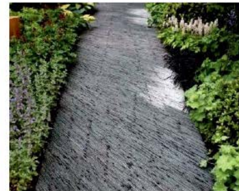
Feature paving patterns Reclaimed clay brick paving Feature clay tiles laid vertically Slate paving laid vertically
