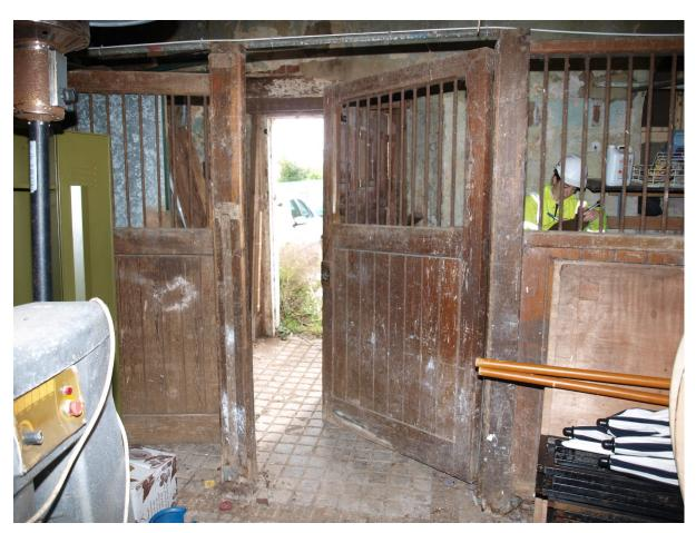
8.11 The width of the stalls may reliably be scaled from the ASE measured drawings, dimensions which will also determine the door and fixed panel widths. The stall side partitions had lower matchboard panels of identical joinery design to the doors but the dowelled metal uprights were shorter, probably about a foot tall, terminating in a narrow timber rail. We know that Room 8 was plastered and the ASE report confirms that walls to the individual stalls were not boarded.
