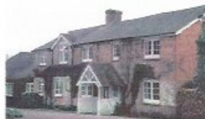
Corner of Church Lane and Houghton Lane, Bury.
